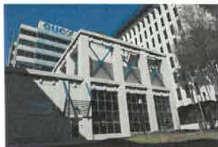
Downtown South Chilled Water Plant
