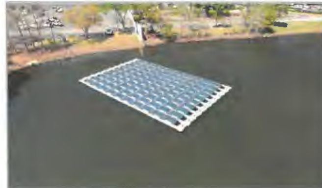
Gardenia Floating Solar
