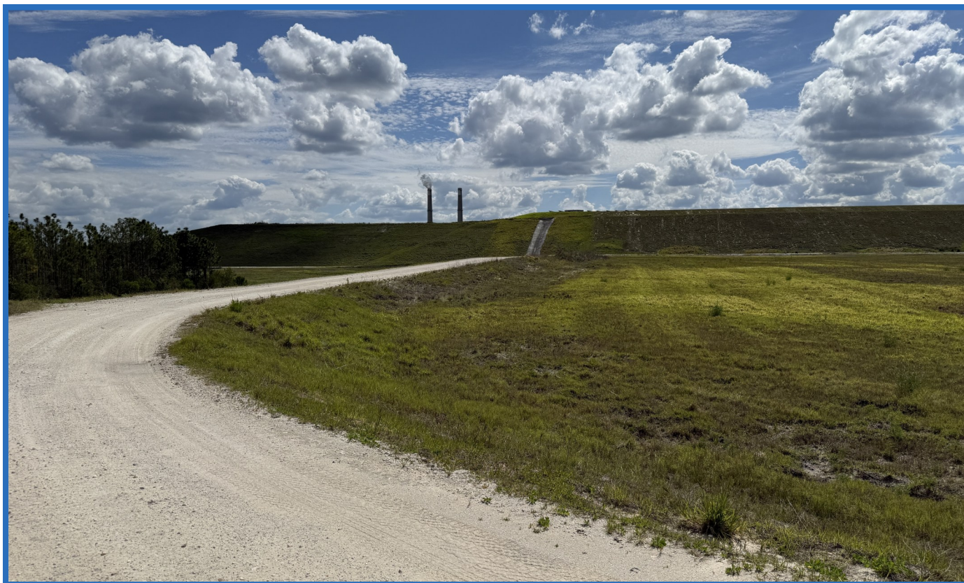
Containment Dike and Northernmost Sub-Cell of Cell 2 (Looking East)
