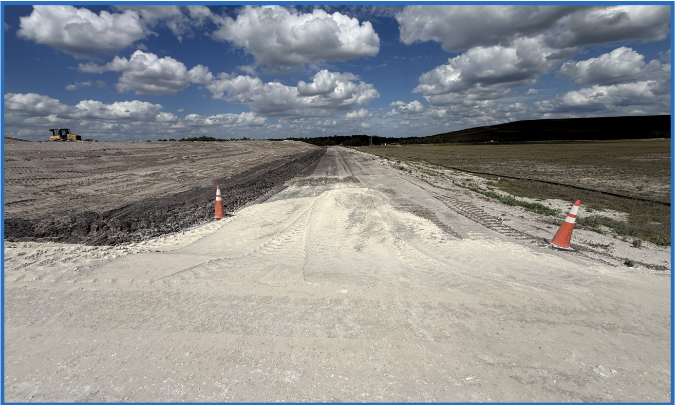
Dike Between Active Sothern Sub-Cells and In-Active Northern Sub-Cells
