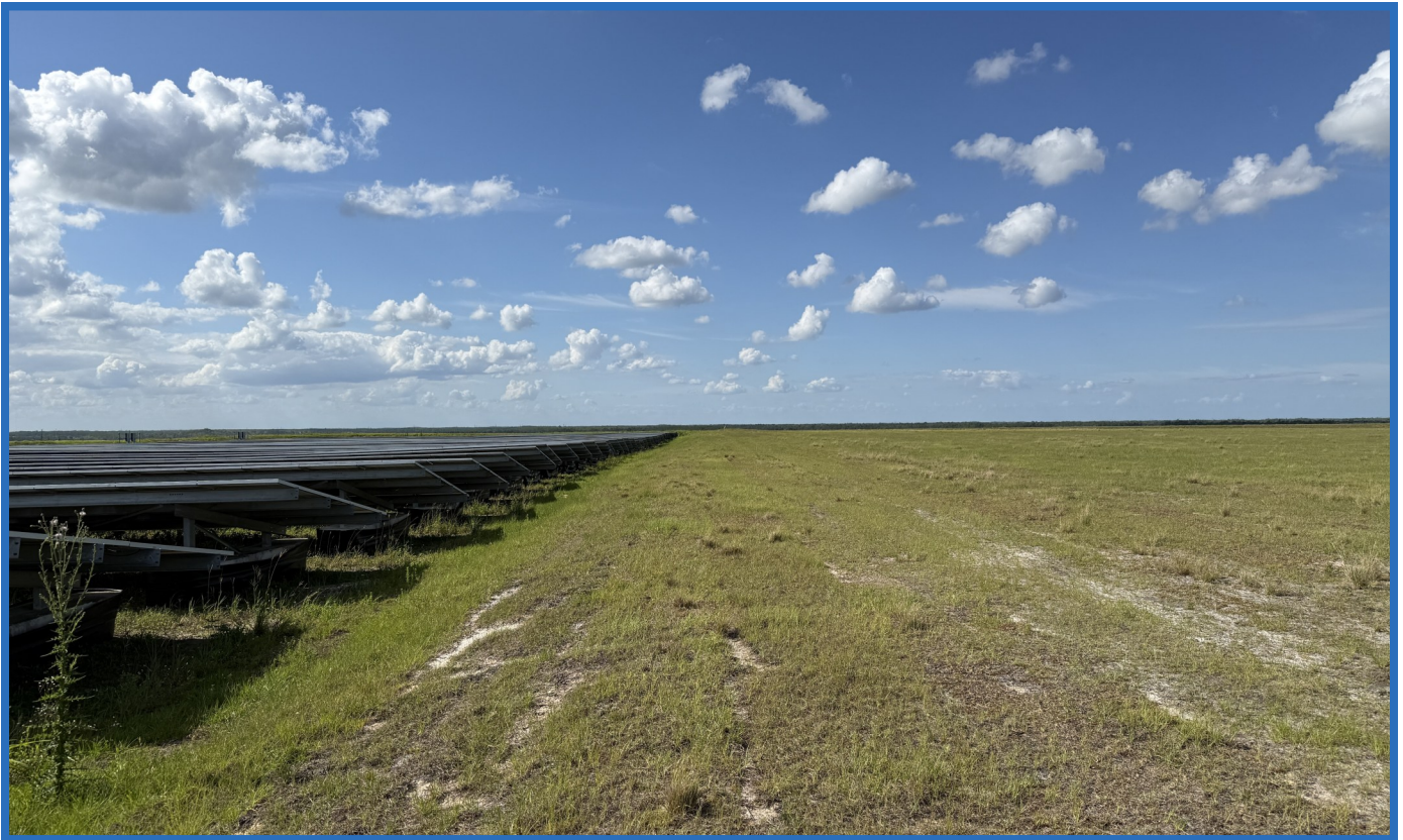
Junction of top of Cell 1 and top of Closed Vertical Expansion (Looking South)
