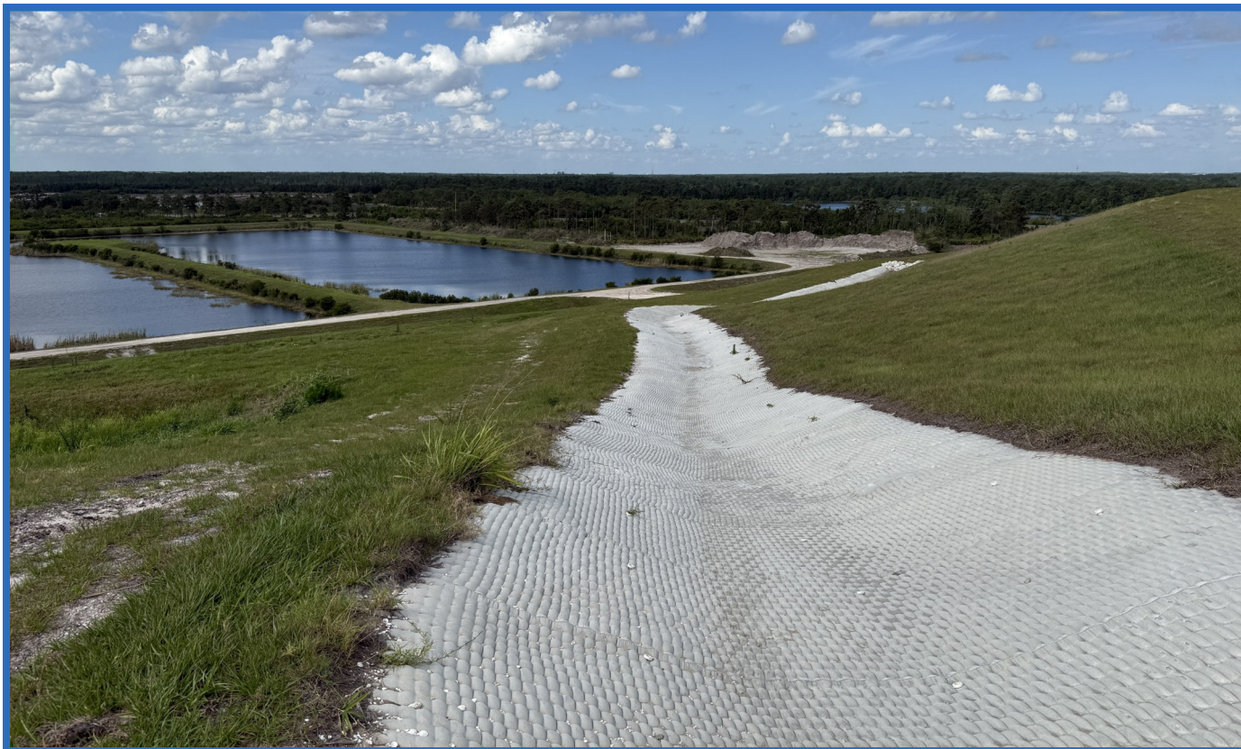
Ramp from Containment Dike of Cell 1 to top of Closed Vertical Expansion of Original CWSA (Looking Southwest from top of the Closed Vertical Expansion of Original CWSA)
