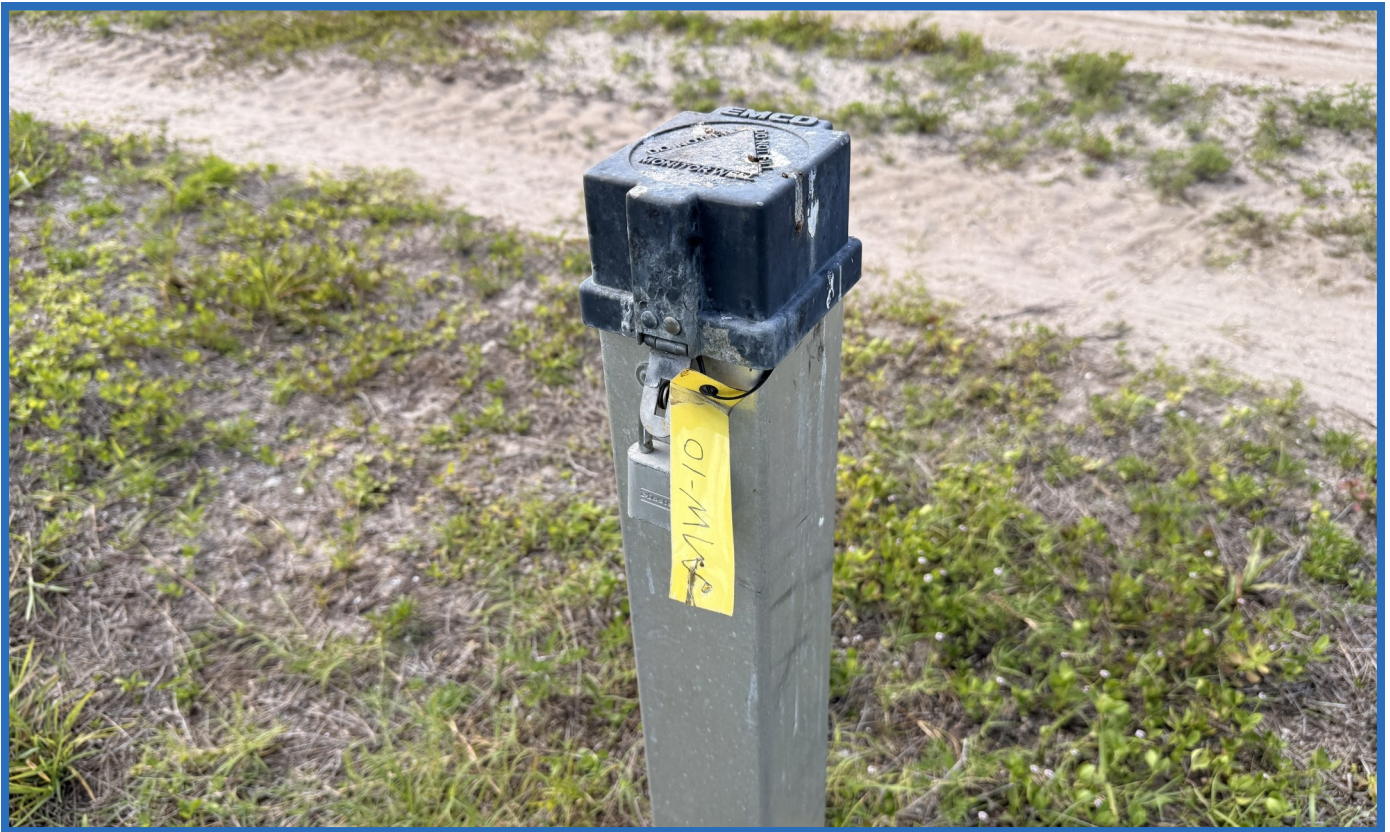
Monitoring Well MW-10 on South Side of Cell 1
