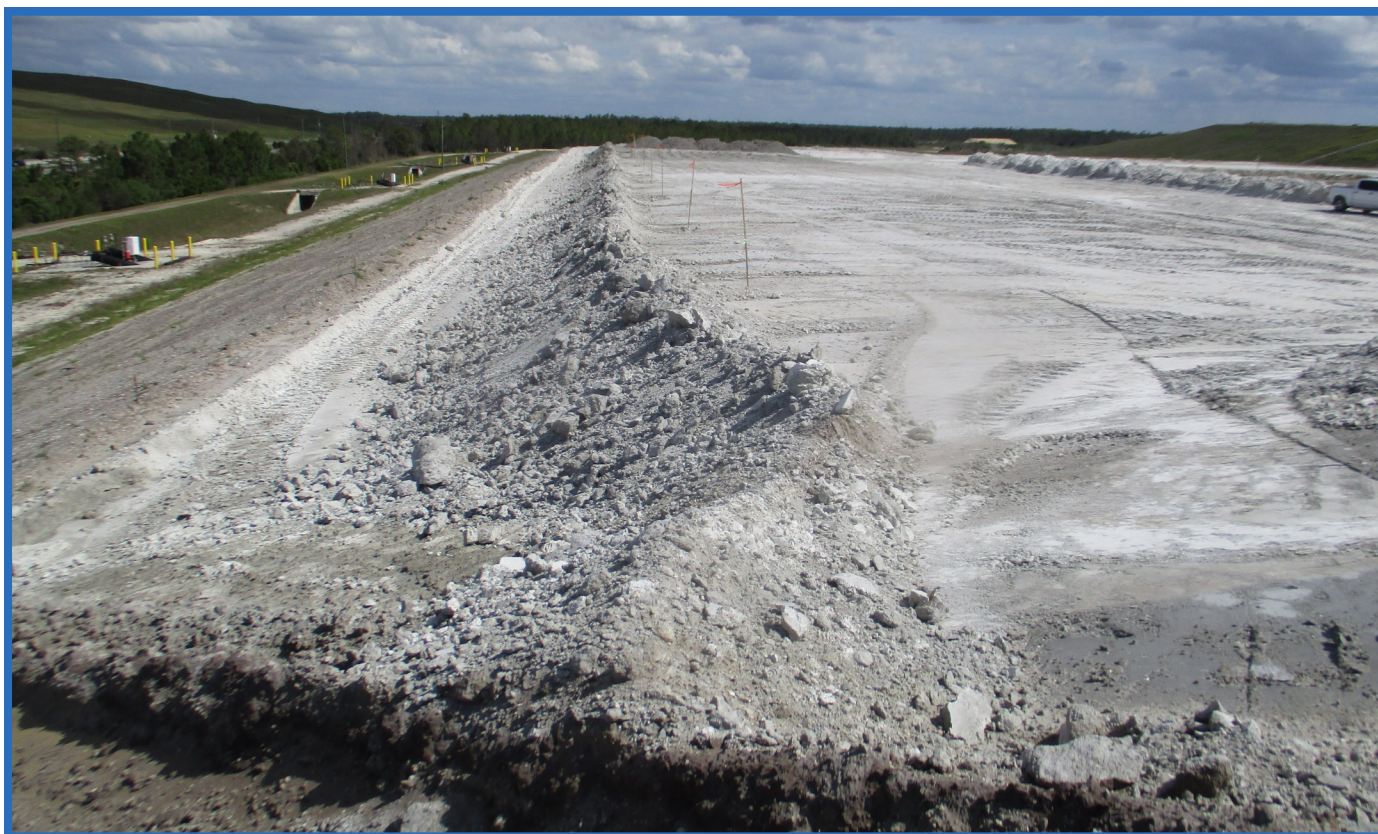
Waste Placed in Two Southern Sub-cells of Cell 2 (Looking Northeast from Southwest Corner of Cell 2)
