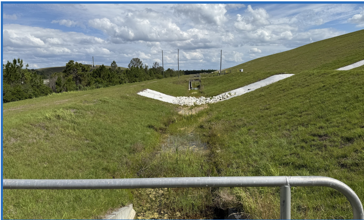
Stormwater Ditch with Box Culverts Between Perimeter Dike and Containment Dike of Cell 1 (Looking North from Perimeter Dike Crossings)
