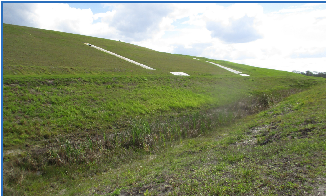
Perimeter Ditch South of Cell 1 (Looking Northeast along South Slope of Cell 1)
