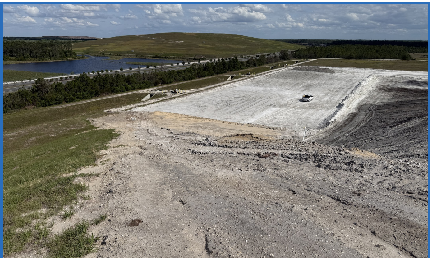
Base of Cell 2 (Looking Northwest from top of North Slope of Cell 1)
