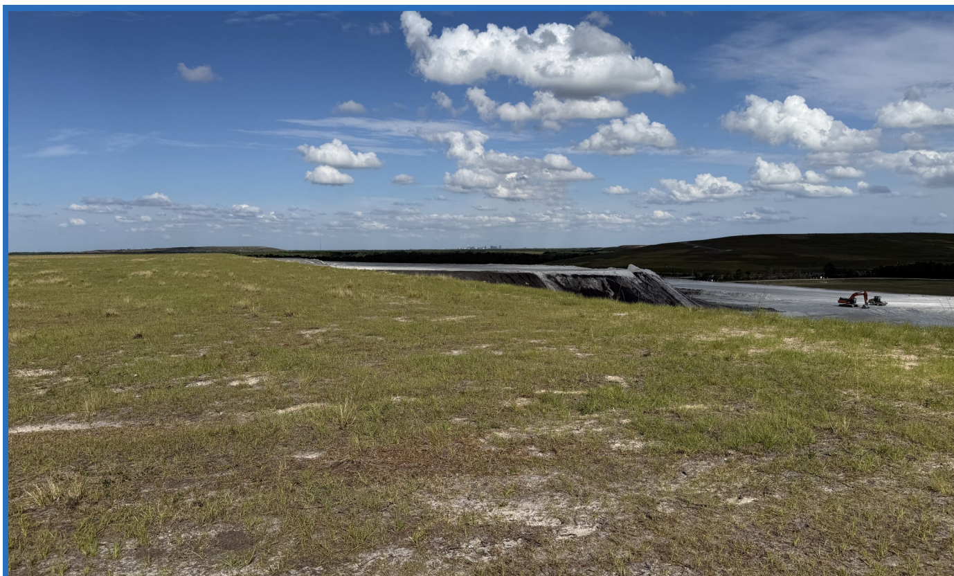
Waste in Cell 2 Abutting Northern Slope of Cell 1 (Looking North from top of the Closed Vertical Expansion of Original CWSA)
