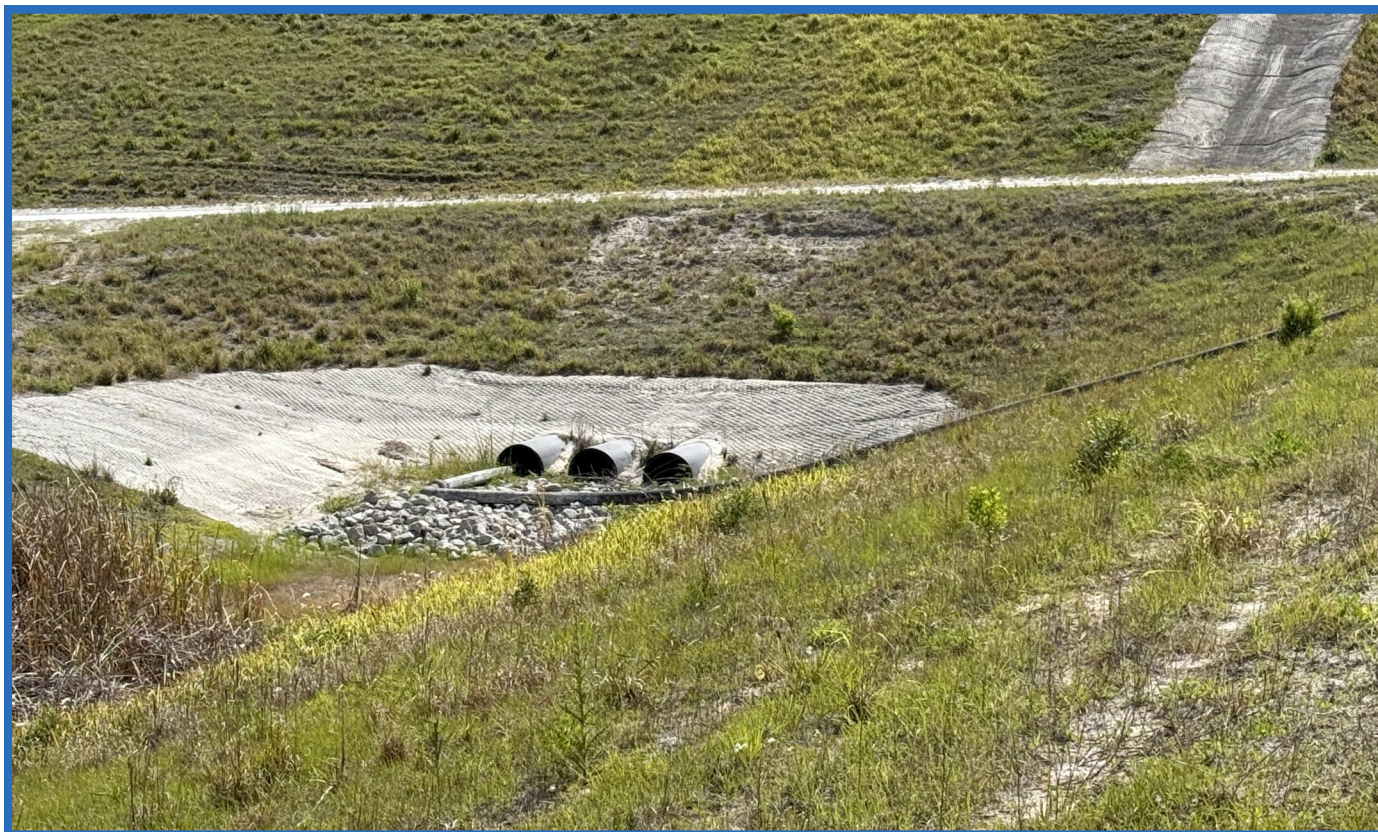
Concrete Flume and HDPE Culverts Draining into Perimeter Ditch on North Side of Cell 2 (Looking East-Northeast)
