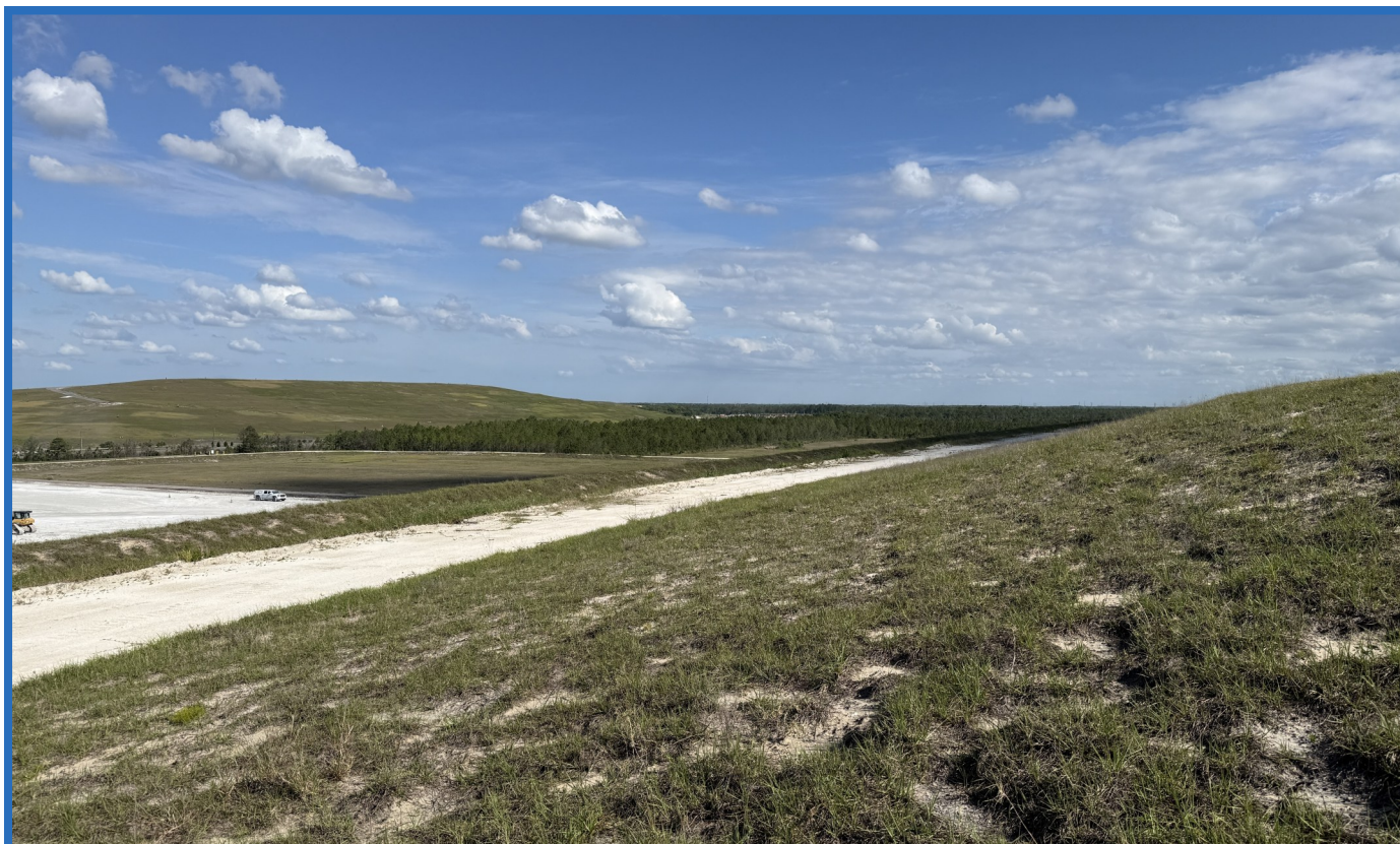
Slope Areas of Cell 2 and two Northern Sub-cells of Cell 2 (Looking North from top of the Closed Vertical Expansion of Original CWSA)
