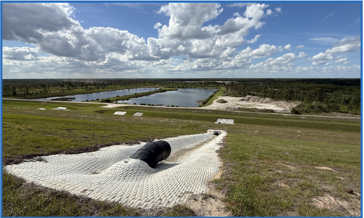
Concrete Flume #3 from top of Cell 1 (Looking South)
