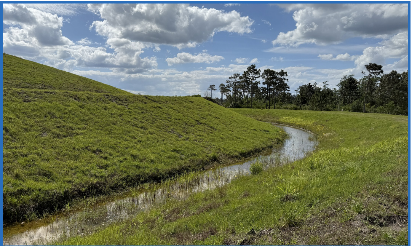
Stormwater Drainage Ditch Between Perimeter Dike and Containment Dike of Cell 1 (Looking Southwest)
