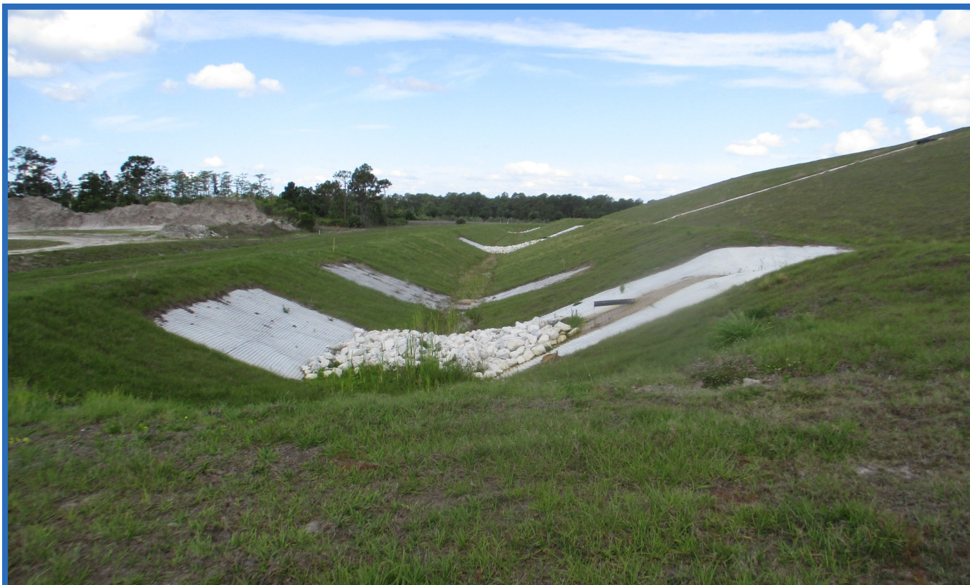
Stormwater Drainage Ditch South of Cell 1 (Looking West)
