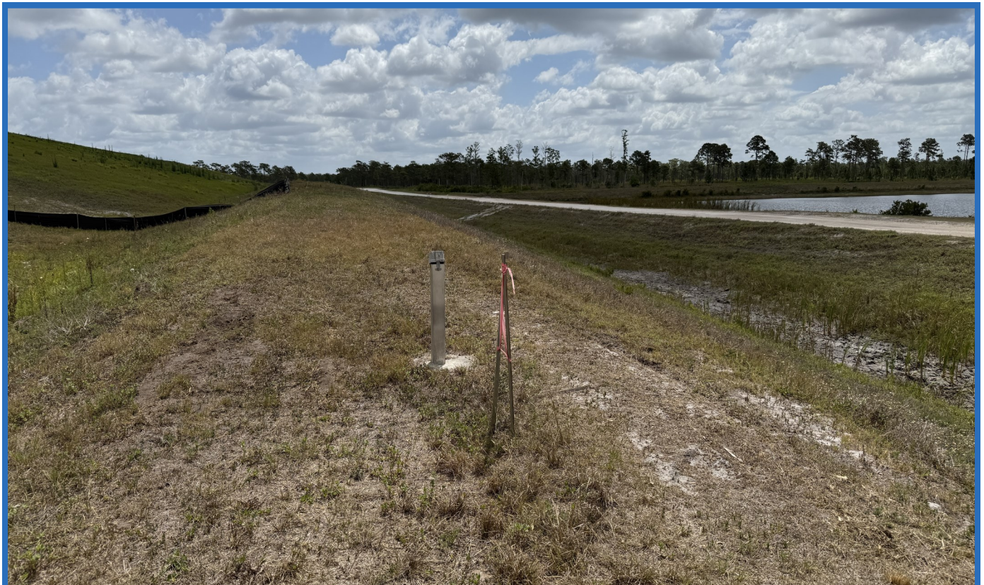
Monitoring Well MW-A on South Side of Cell 1
