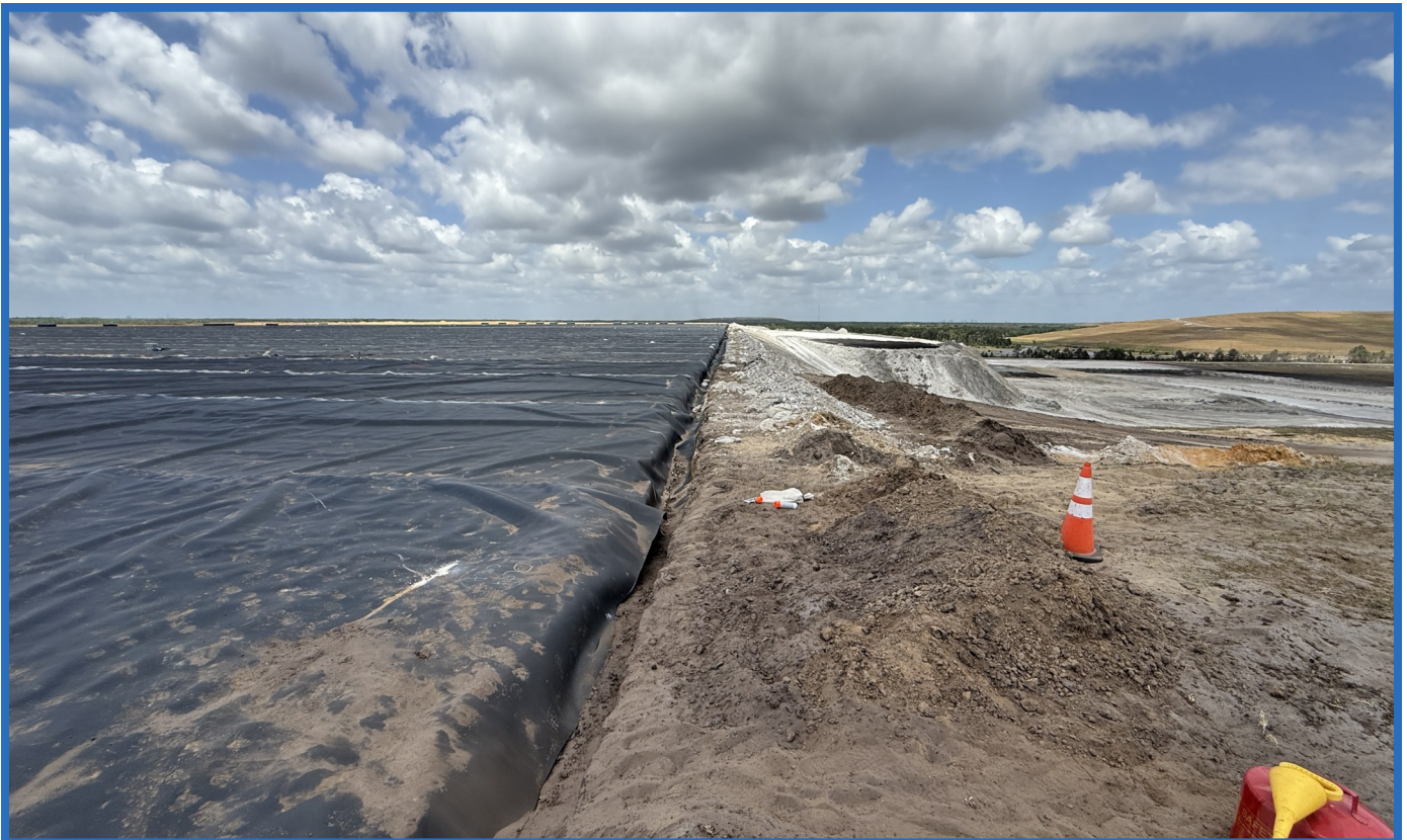
North Anchor Trench of Closure Liner atop Cell 1, Waste in Cell 2 Abutting Northern Slope of Cell 1 (Looking North from top of the Closed Vertical Expansion of Original CWSA)
