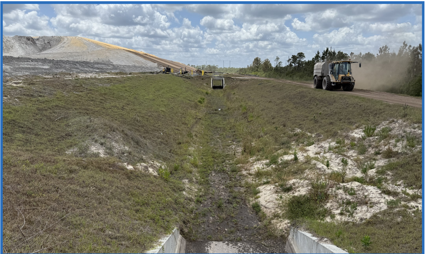
Stormwater Ditch with Box Culverts Between Perimeter Dike and Containment Dike of Cell 2 (Looking South from Perimeter Dike Crossings)
