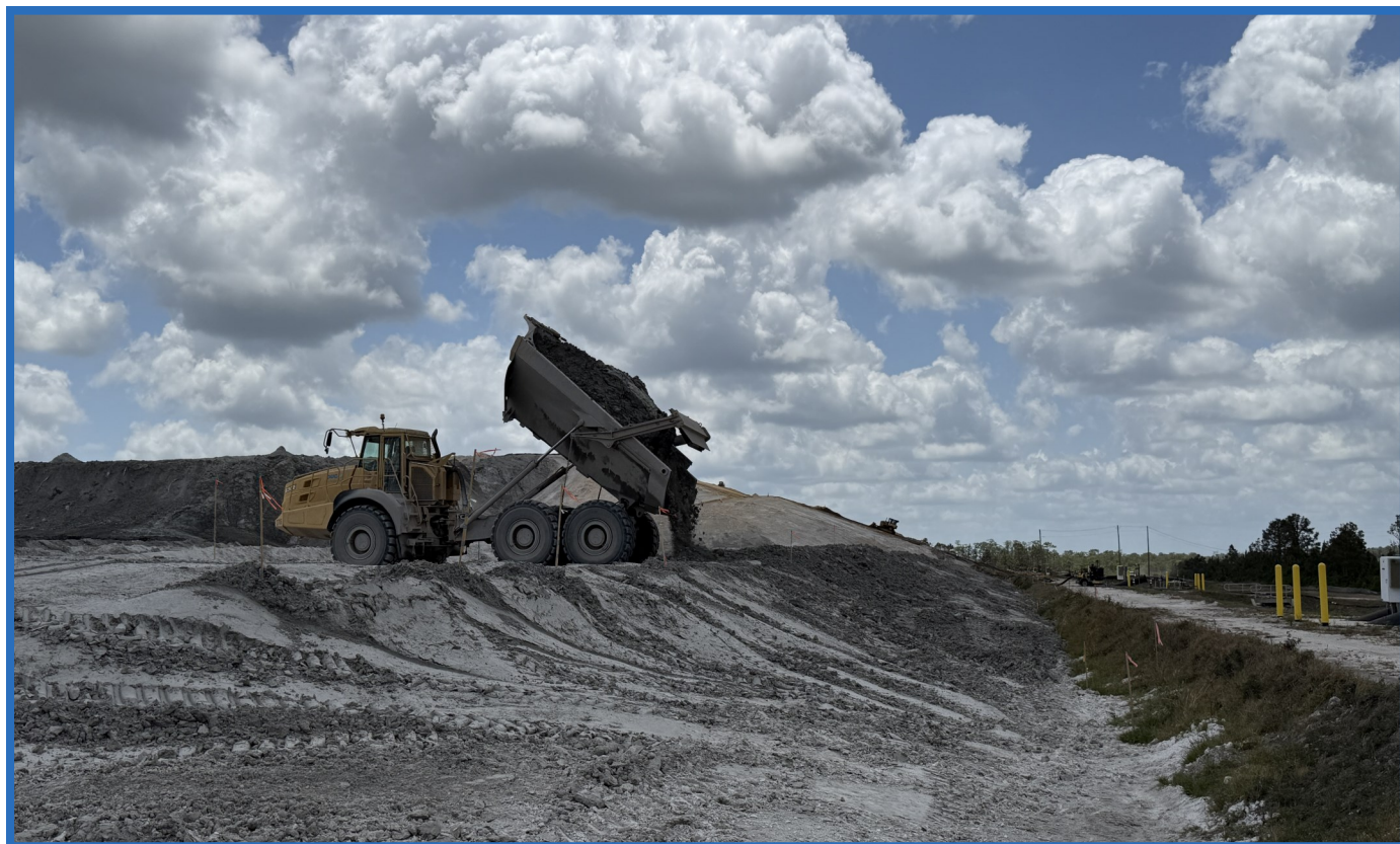
Articulated Dump Truck Placing Waste in Cell 2 (Looking South/Southeast)
