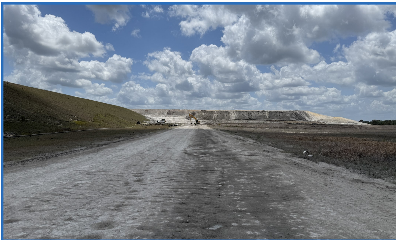
Access Road through Bottom of Cell 2 (Looking South)
