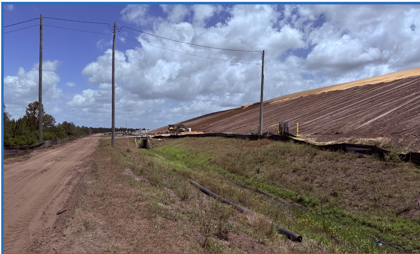
Stormwater Ditch Between Perimeter Dike and Containment Dike of Cell 1 Undergoing Closure (Looking North from Perimeter Dike)
