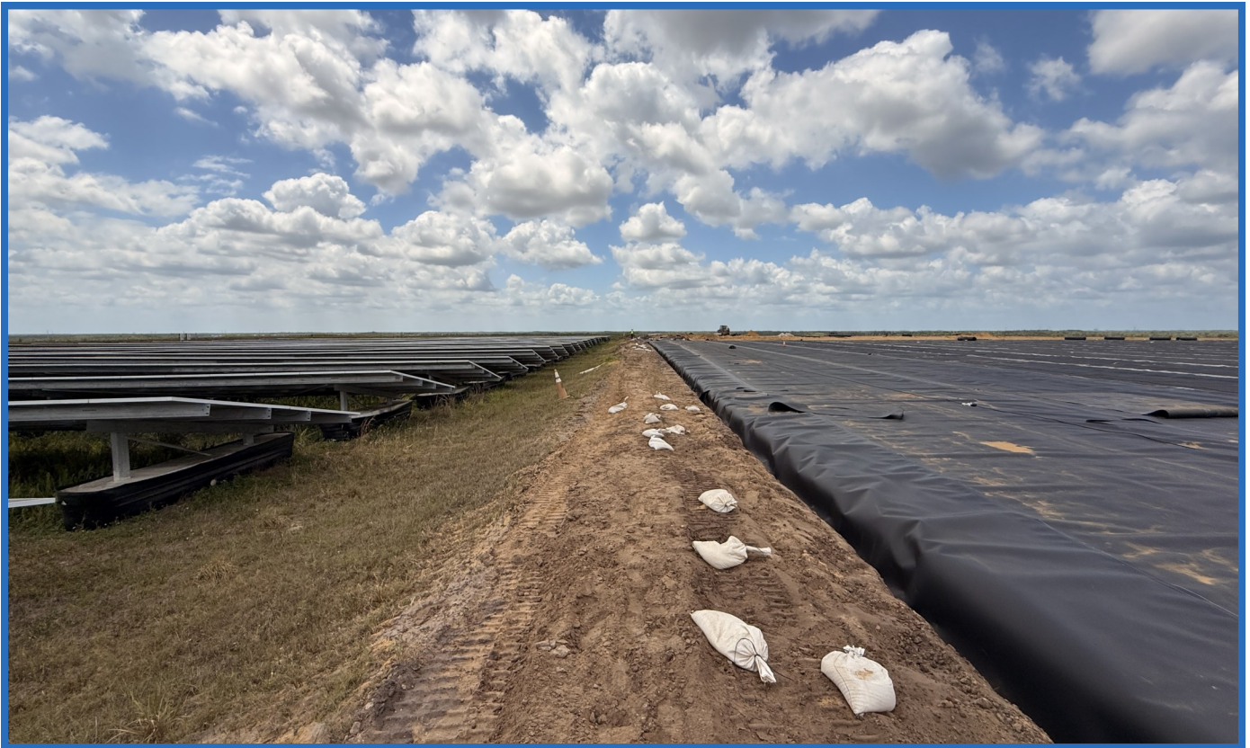
East Anchor Trench of Closure Liner atop Cell 1 (Looking South from top of the Closed Vertical Expansion of Original CWSA)
