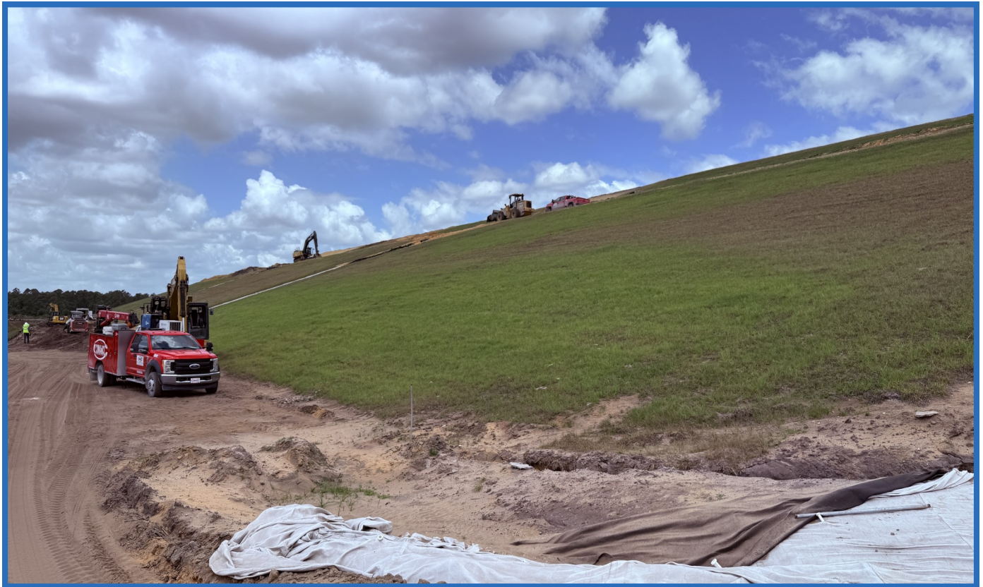
Sod on Lower Slopes on Cell 1 Currently Undergoing Closure (Looking Northwest from Containment Dike on South of Cell 1)
