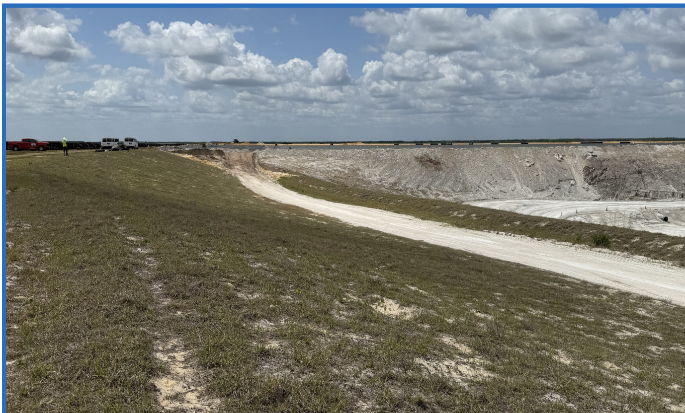
Junction of Waste Mound in Cell 1 with Cell 2, abutting the western slope of Original CWSA (Looking South from top of the Closed Vertical Expansion of Original CWSA)
