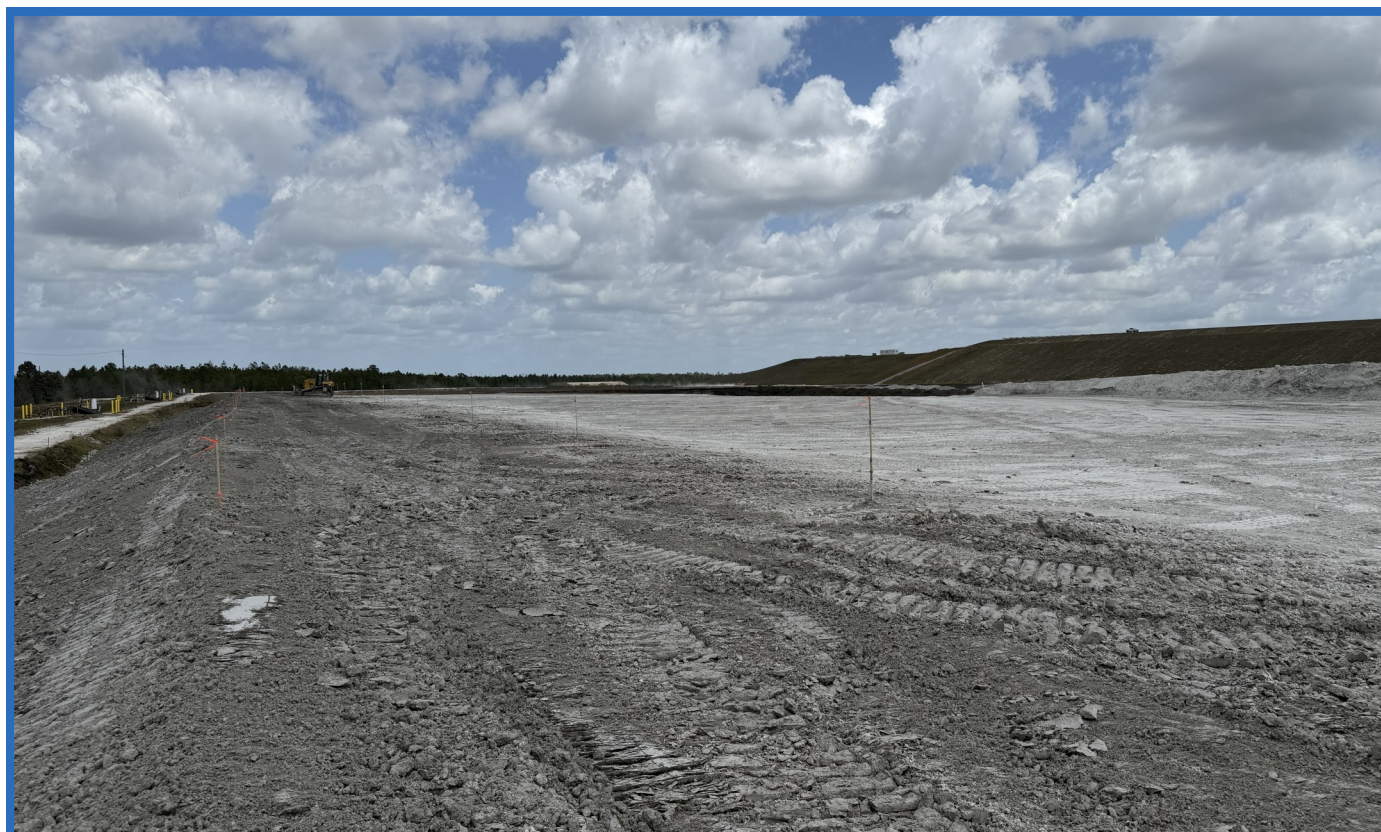
Waste Placed in Two Southern Sub-cells of Cell 2 (Looking Northeast from Southwest Corner of Bottom of Cell 2)
