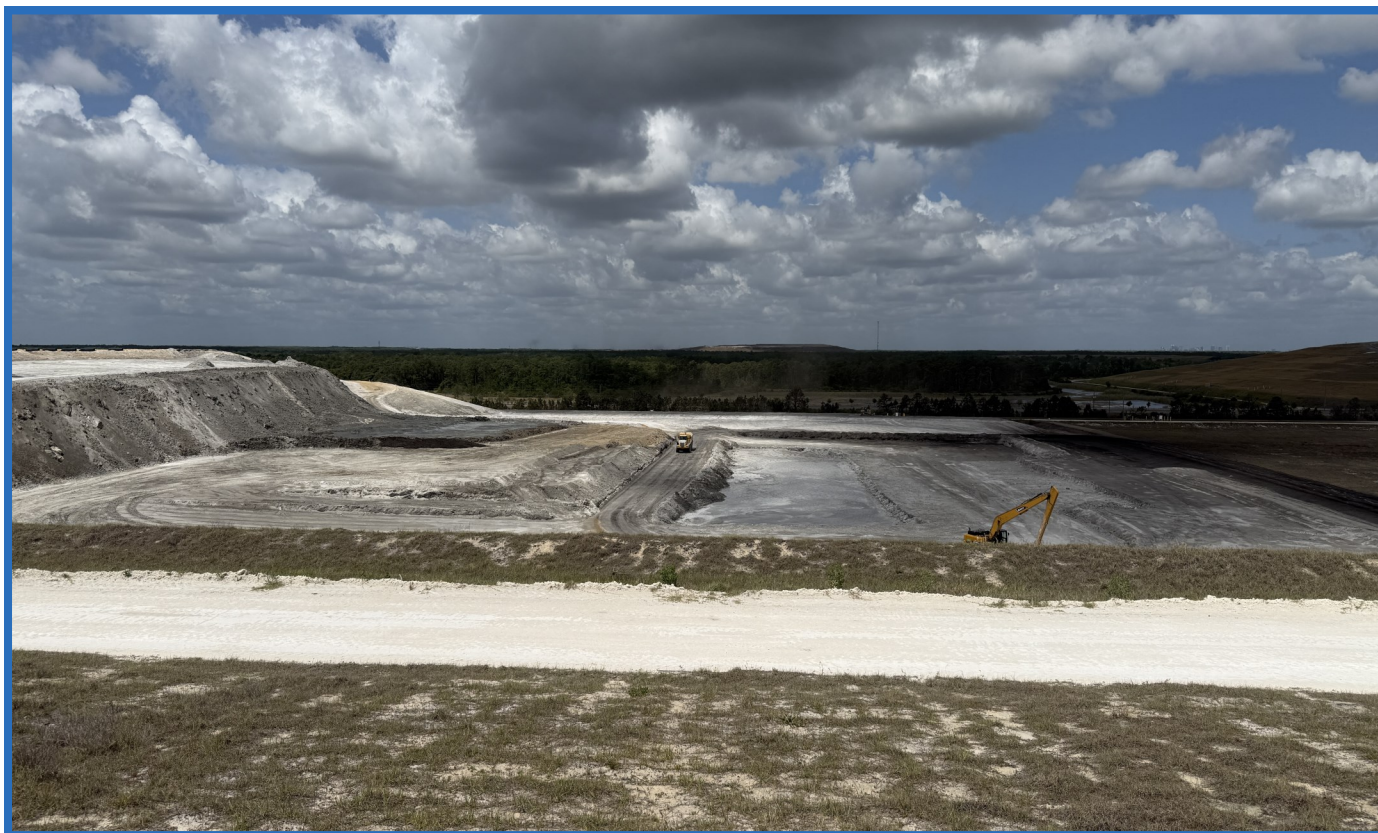
Waste Placed in Cell 2 bottom and slope areas (Looking West from top of the Closed Vertical Expansion of Original CWSA)
