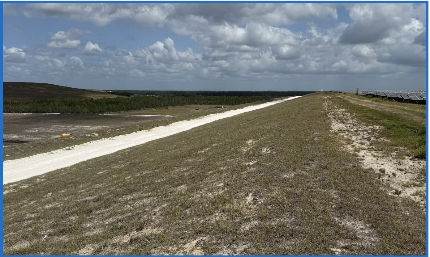
Slope Areas of Cell 2 and two Southern Sub-cells of Cell 2 (Looking North from top of the Closed Vertical Expansion of Original CWSA)
