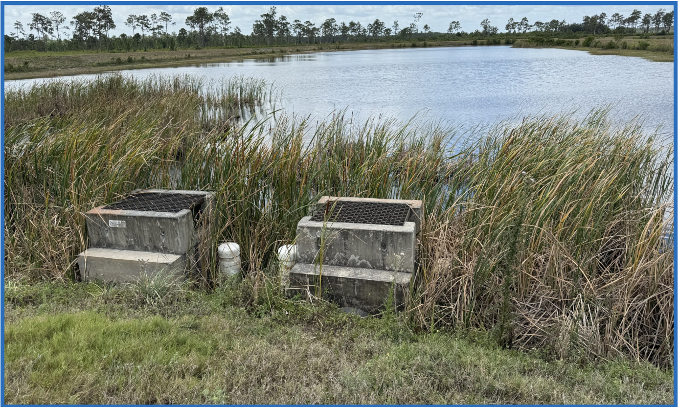
Discharge Structures for Wet Detention Pond (Looking South-Southeast)
