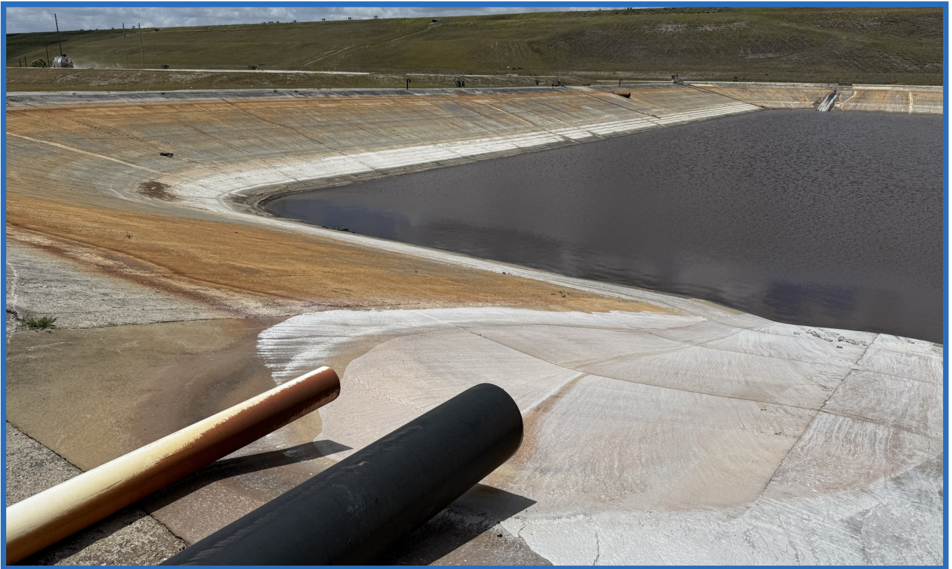
Southern Compartment of CWSA Runoff Pond (Looking Southwest/West)
