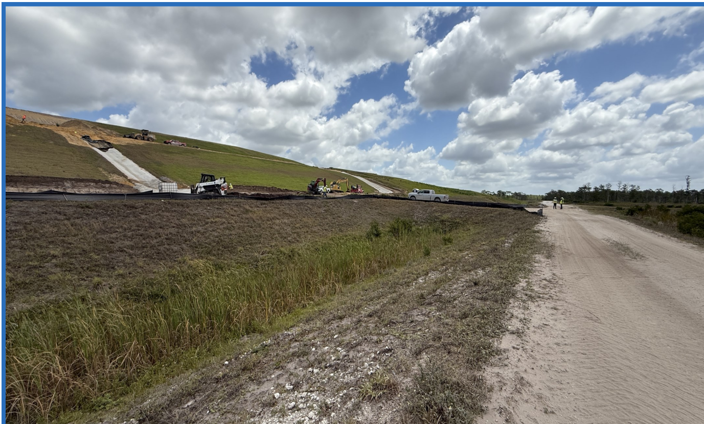
Perimeter Ditch South of Cell 1 (Looking Northeast towards South Slope of Cell 1 Undergoing Closure)
