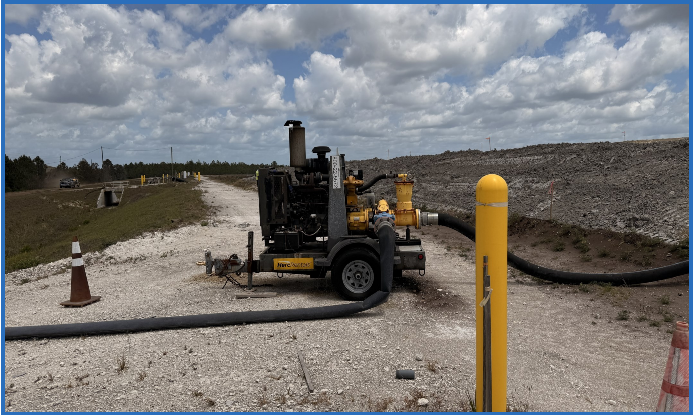
Diesel Auxiliary Pump with Intake Deployed in Cell 2, Sub-cell A (Looking North)
