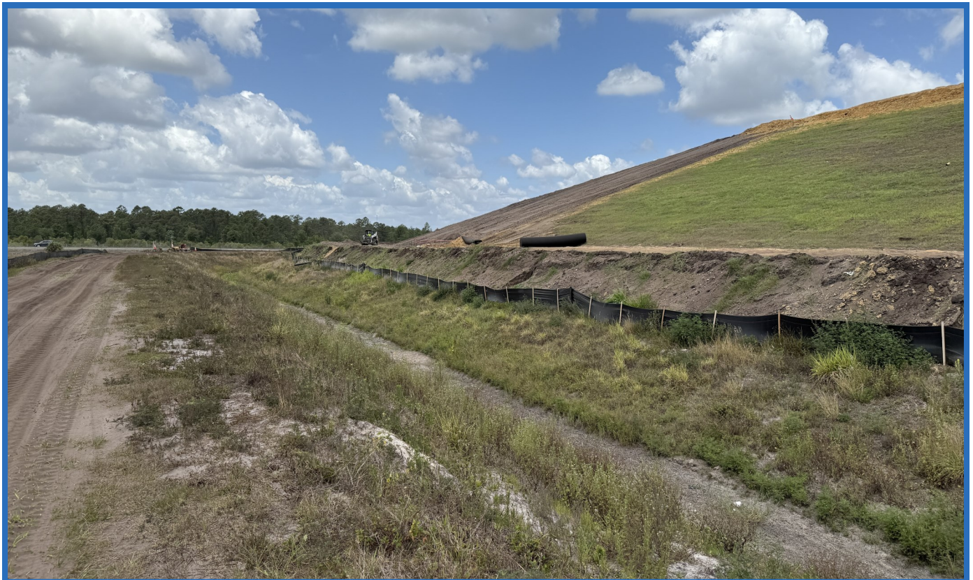
Stormwater Ditch Between Perimeter Dike and Containment Dike of Cell 1 Under- going Closure (Looking East from Perimeter Dike)
