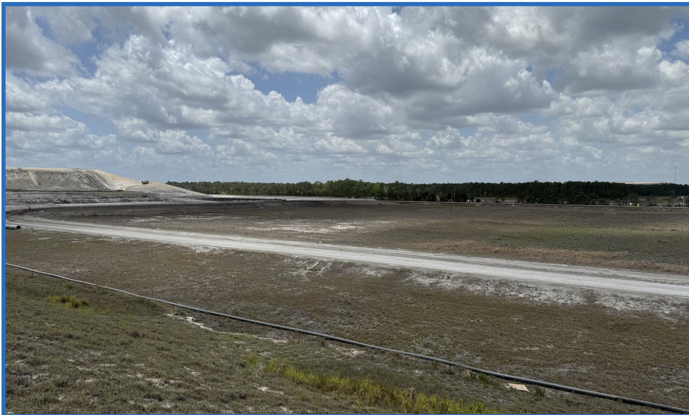
Two Northern Sub-Cells of Cell 2, Which are not receiving Waste (Looking Southwest from top of the Closed Vertical Expansion of Original CWSA)
