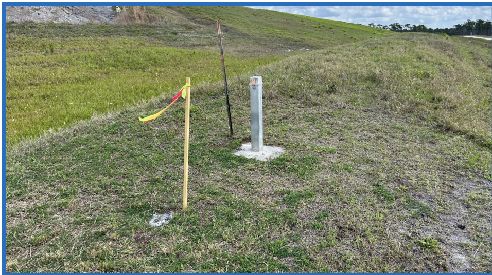
Monitoring Well MW-A on Southern Side of Cell 1
