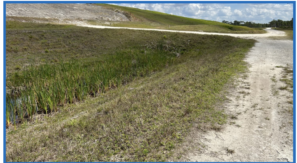
Perimeter Ditch and Culvert Under Access Ramp Crossing Ditch, Looking Northeast Toward Southern Slope of Waste Mound in Cell 1
