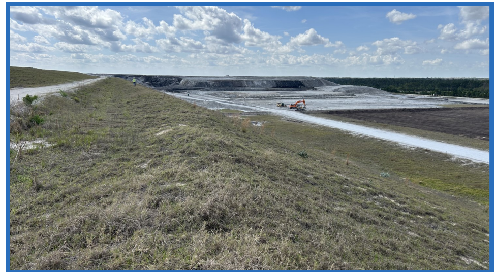
Bench on Closed Vertical Expansion and Side Slope of Cell 2, Looking Southwest Toward Cell 1
