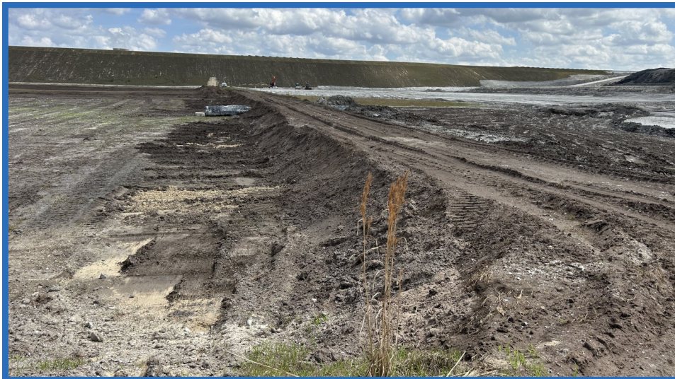
Earthen Dike/Road Between Subcells 2 and 3 of Cell 2, Looking Southeast
