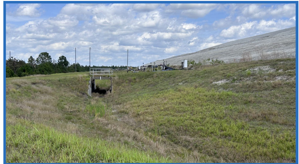
Box Culvert in Perimeter Ditch at Southwestern Corner of Cell 1, Looking North
