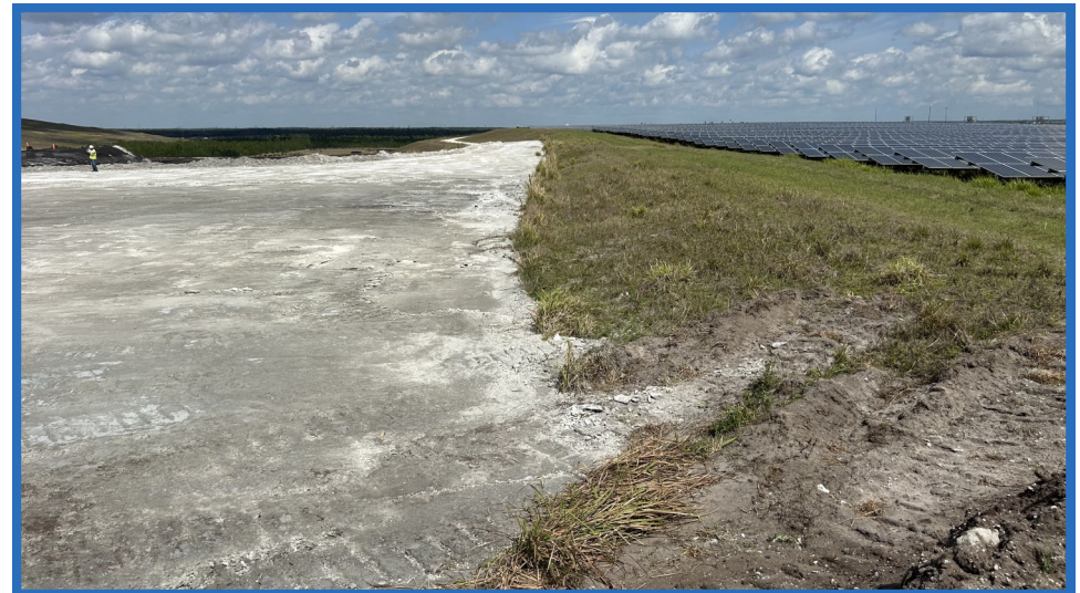
Top of Waste in Cell 1 and Photovoltaic Solar Panels on Top of Closed Vertical Expansion of Original CWSA, Looking Northeast
