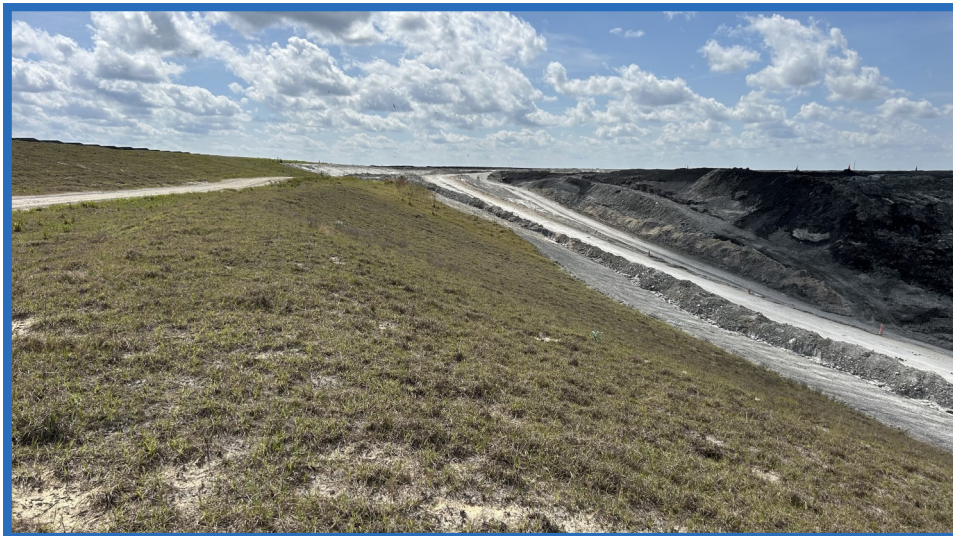
Junction of Waste Mound in Cell 1 with Cell 2 and Reverse Bench of Closed Vertical Expansion of Original CWSA, Looking Southeast
