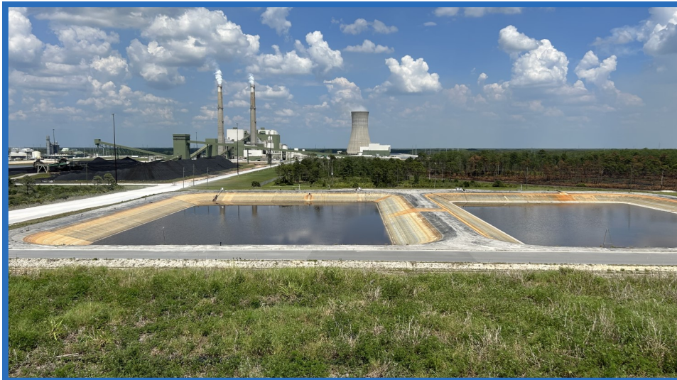
CWSA Runoff Pond, Looking East
