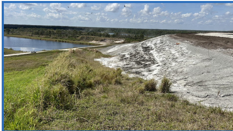
Wet Detention Pond, Looking Southwest from Bench at Juncture with Closed Original CWSA
