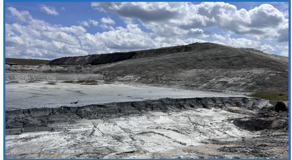
Northern Slope and Northwestern Corner of Waste Mound in Cell 1, and Waste in Subcell 1 of Cell 2, Looking Southeast
