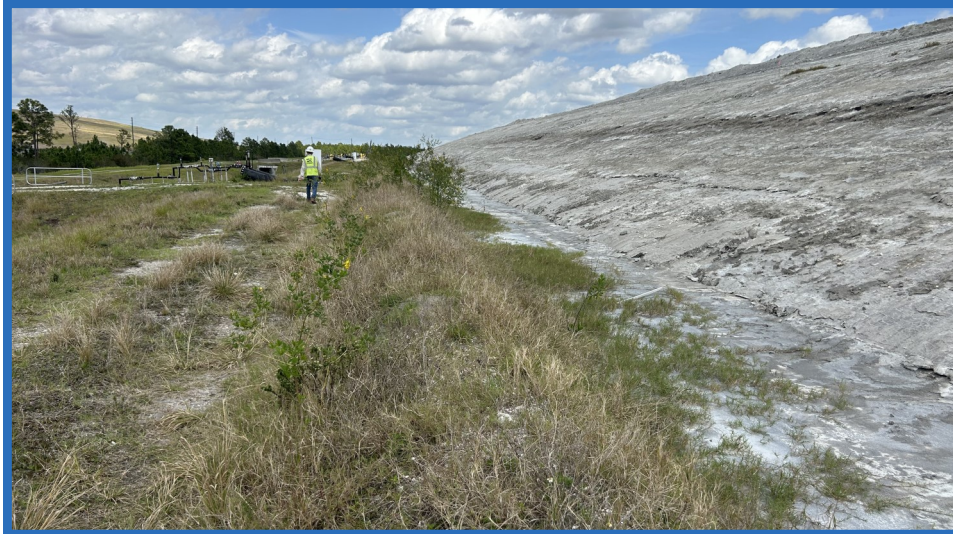
Western Slope of Waste Mound in Cell 1, Looking North
