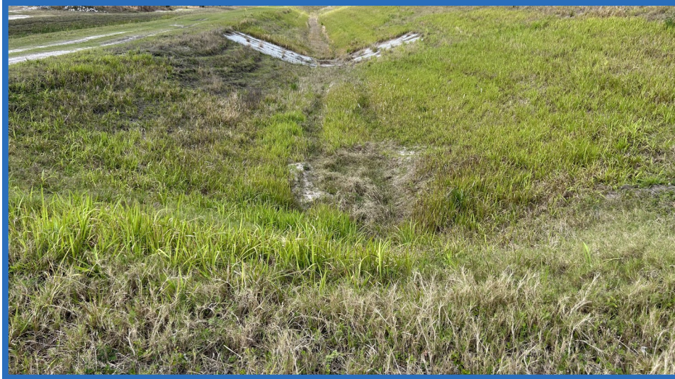
Perimeter Dike/Road and Ditch South of Cell 1, Looking West from Access Road Crossing Ditch
