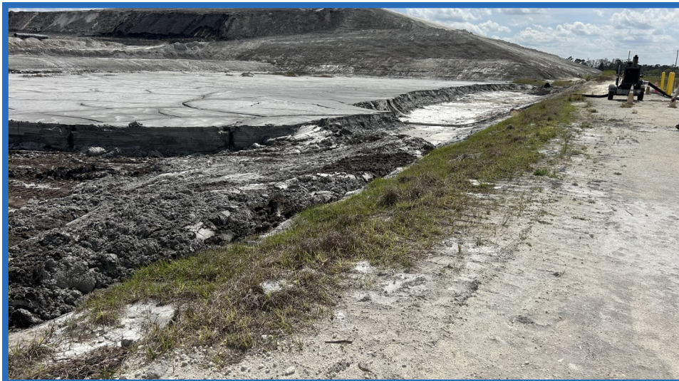
Waste Placed in Subcell 1 of Cell 2 and Diesel Auxiliary Pump with Intake Deployed in Cell 2, Looking South-Southeast
