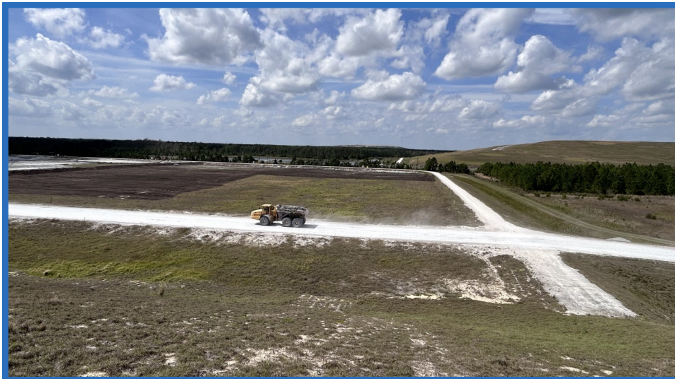
Articulated Dump Truck Hauling ProMat on Access Road through Cell 2, Looking West
