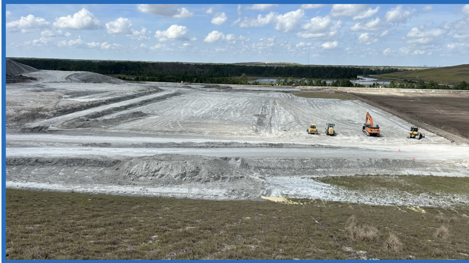
Waste Placed in Cell 2 and Northern Slope of Waste Mound in Cell 1, Looking West from Reverse Bench of Closed Vertical Expansion of Original CWSA
