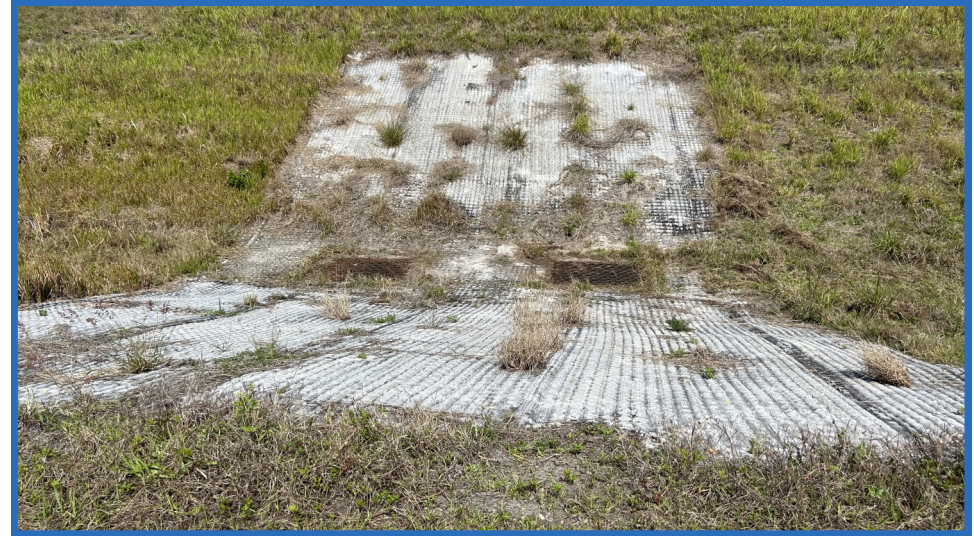
Fabriform with Inlets to Wet Detention Pond in Perimeter Ditch in Southwestern Part of Cell 1, Looking North
