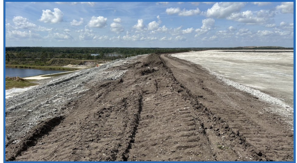
Top of Waste in Cell 1, Looking West from Reverse Bench of Closed Vertical Expansion of Original CWSA
