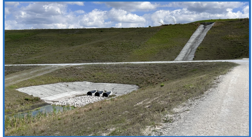
Concrete Flume and HDPE Culverts Draining into Perimeter Ditch on North Side of Cell 2, Looking East-Northeast
