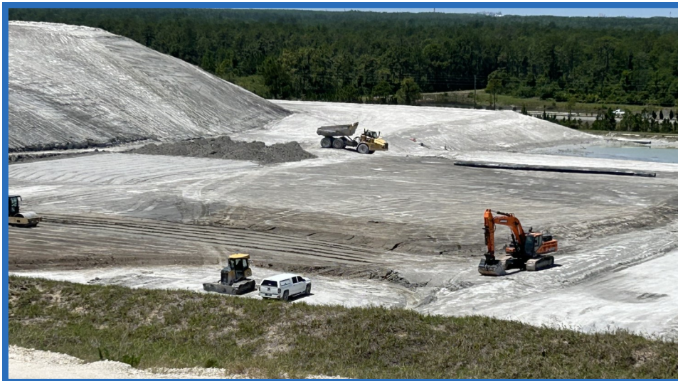
Articulated Dump Truck Depositing Waste in Cell 2, Looking West
