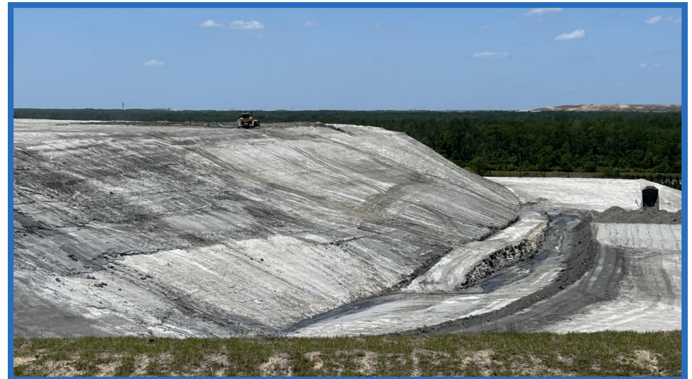
Spreading Waste with Dozer on Top of Cell 1
