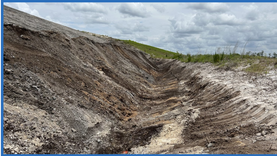
Re-graded Waste on South Side of Cell 1, Looking East
