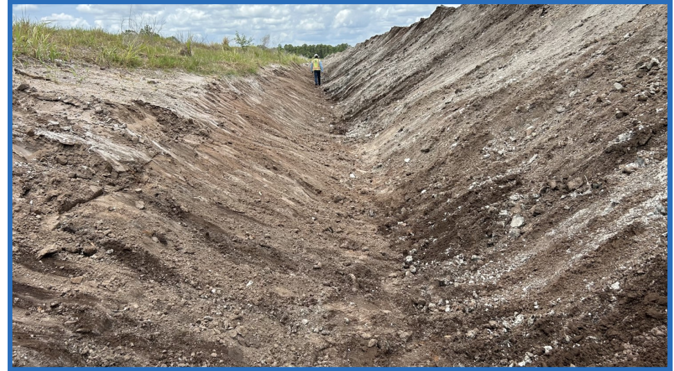
Re-graded Waste on South Side of Cell 1, Looking West
