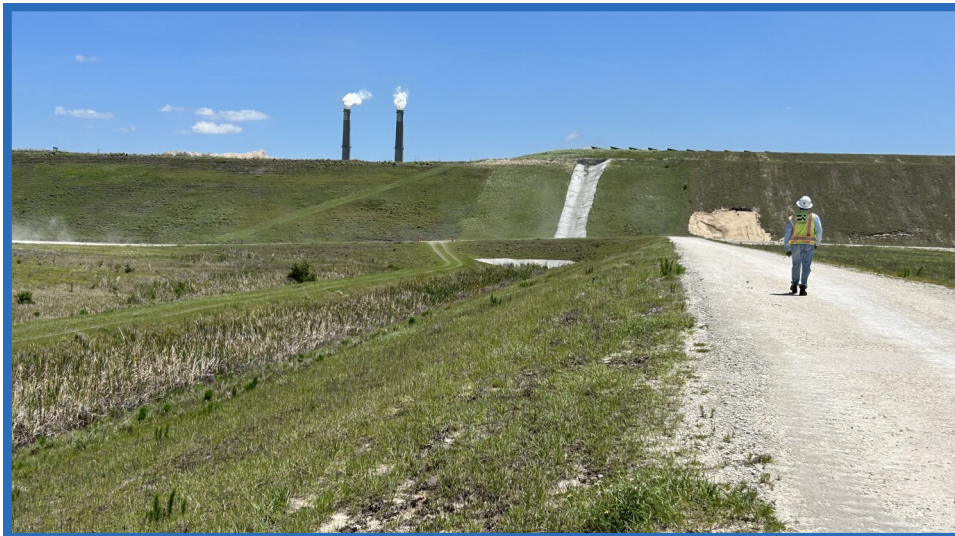
Containment Dike and Perimeter Ditch on North Side of Cell 2, Looking East
