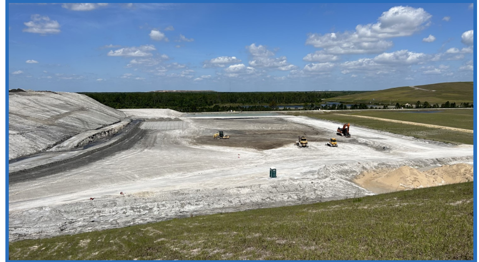
Waste Placement in Cell 2 and Northern Slope of Waste Mound in Cell 1, Looking West
