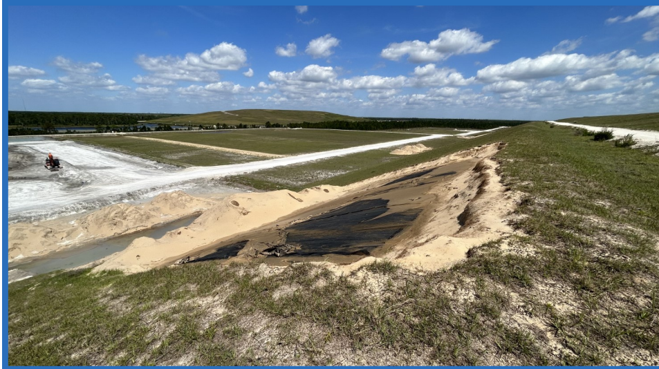
Cell 2, Looking Northwest from Reverse Bench of Closed Vertical Expansion of Original CWSA
