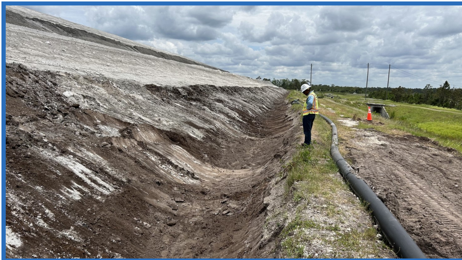
Re-graded Waste on West Side of Cell 1, Looking South
