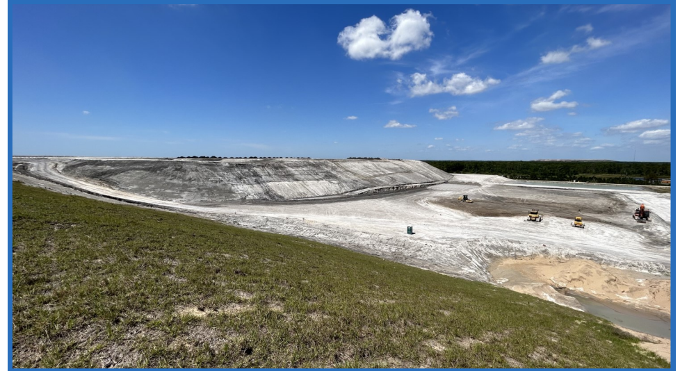
Access Ramp from West Haul Road Through Cell 2 to Top of Cell 1, Looking Southwest
