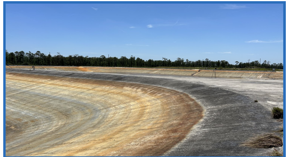
Divider Dike Between CWSA Runoff Pond North and South Compartments, Looking East-Southeast
