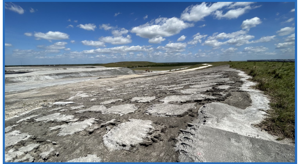
Top of Waste in Cell 1, Looking North-Northwest from Reverse Bench of Closed Vertical Expansion of Original CWSA
