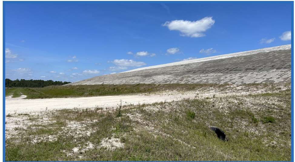
Culvert Under Access Ramp Crossing Ditch, Looking Northwest Toward Southern Slope of Waste Mound in Cell 1
