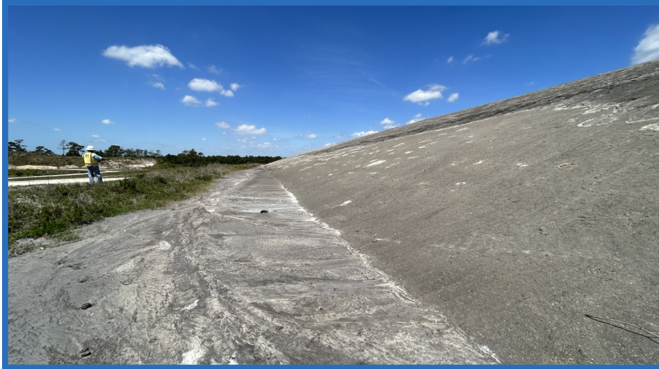
Southern Slope of Waste Mound in Cell 1, Looking South
