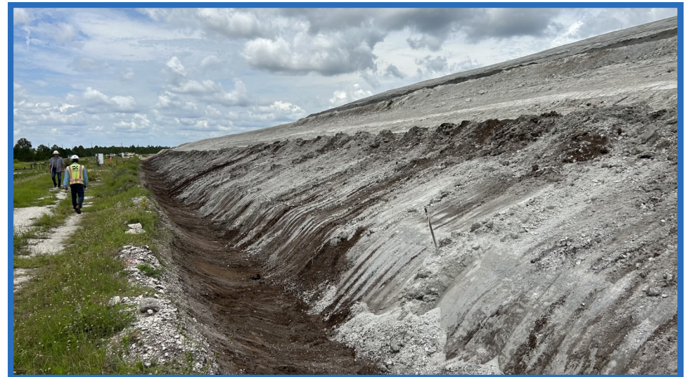
Re-graded Waste on West Side of Cell 1, Looking North
