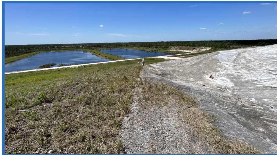
Wet Detention Pond, Looking Southwest from Top of Cell 1 at Juncture with Closed Original CWSA
