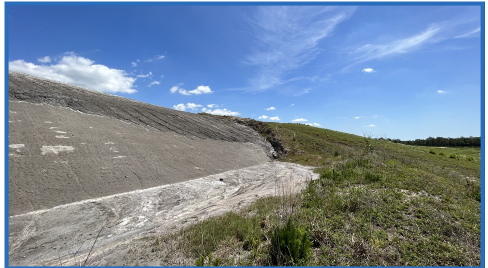
Southern Slope of Waste Mound, in Cell 1 Where It Abuts Closed Original CWSA, Looking Northeast
