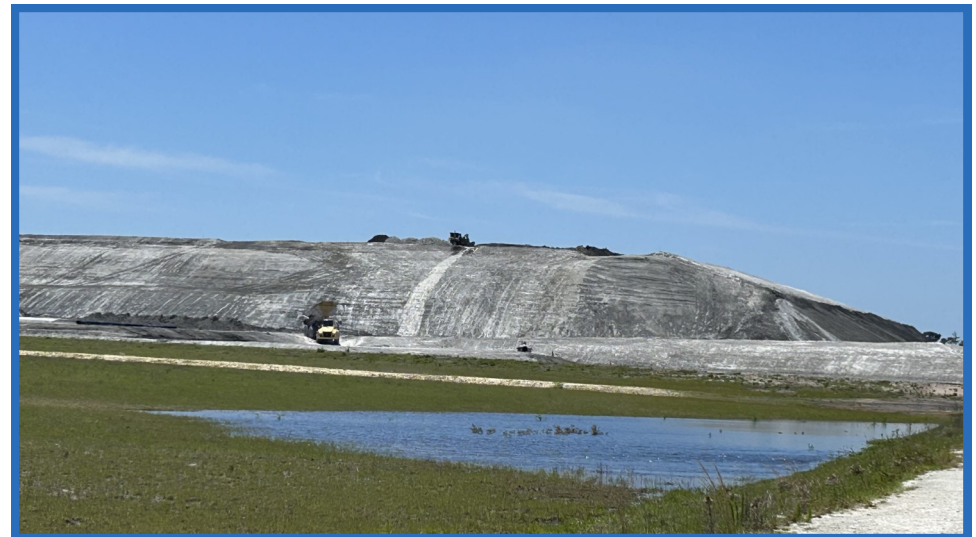
Northern Slope of Waste Mound in Cell 1, Looking South
