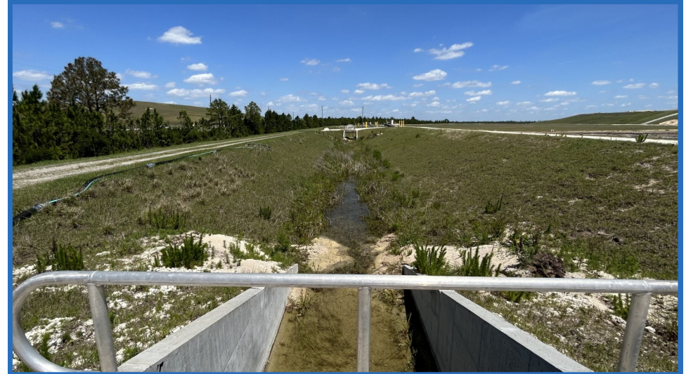
Perimeter Ditch West of Cell 2, Looking North from Box Culvert Crossing
