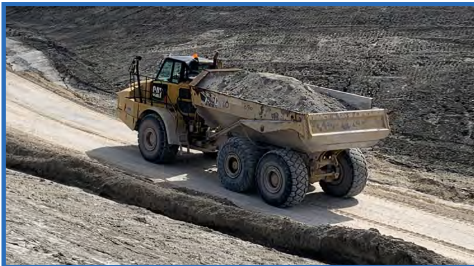
Articulated Dump Truck Hauling Waste Up Access Road to Western Slope of Closed Original CWSA
