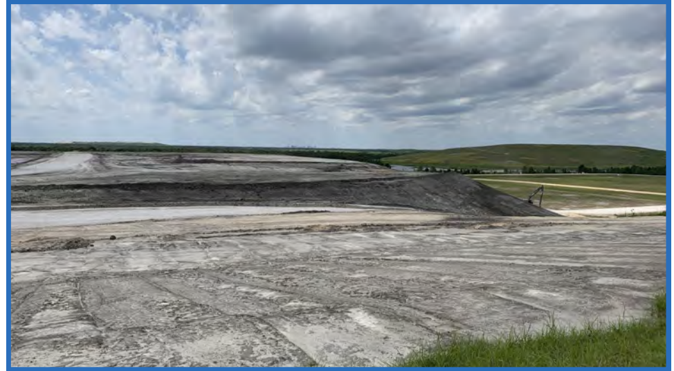
Top of Waste in Cell 1, Looking West-Northwest from Reverse Bench of Closed Vertical Expansion of Original CWSA
