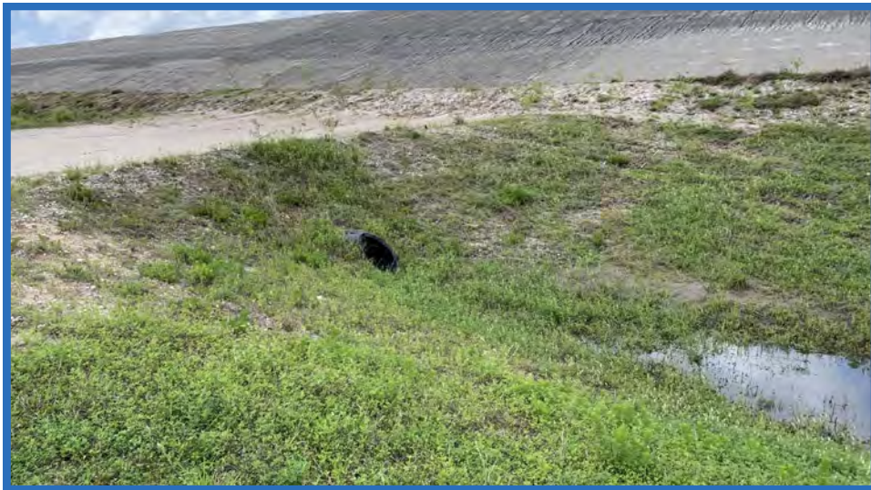
Culvert Under Access Ramp Crossing Ditch, Looking Northwest Toward Southern Slope of Waste Mound in Cell 1
