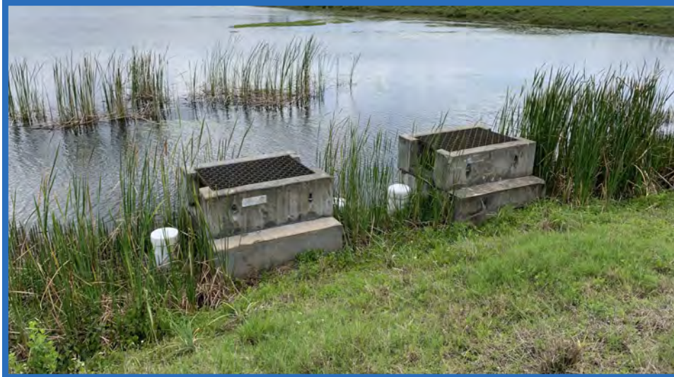
Discharge Structures for Wet Detention Pond, Looking Southwest
