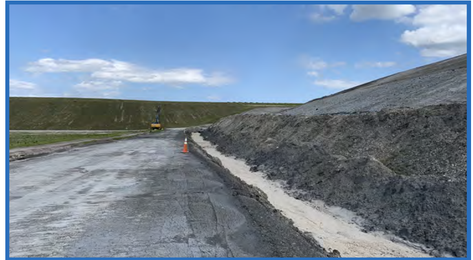
Northern Slope of Waste Mound in Cell 1 and Containment Dike Between Cell 1 and Cell 2, Looking East
