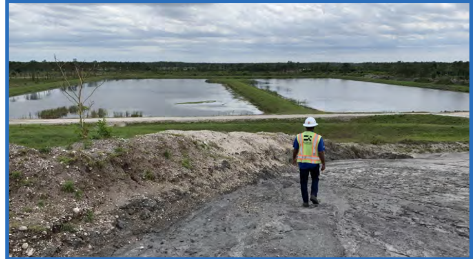
Wet Detention Pond, Looking South from Cell 1
