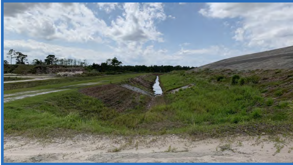
Perimeter Road and Ditch South of Cell 1, Looking West from Access Road Crossing Ditch
