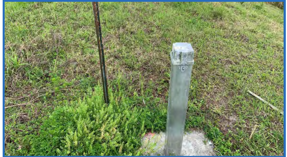
Monitoring Well MW-A on Southern Side of Cell 1, Looking East
