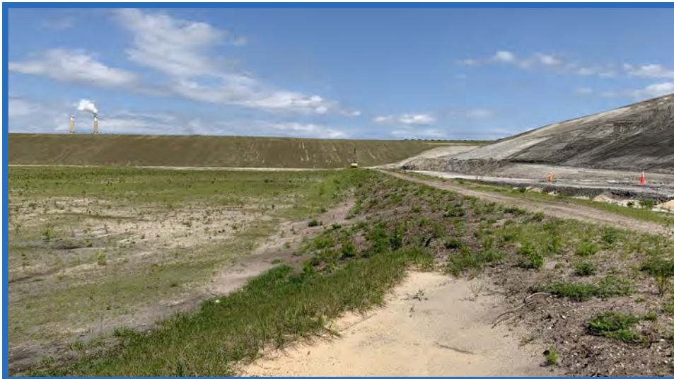
Containment Dike Between Cell 1 (Right) and Cell 2 (Left), Looking East
