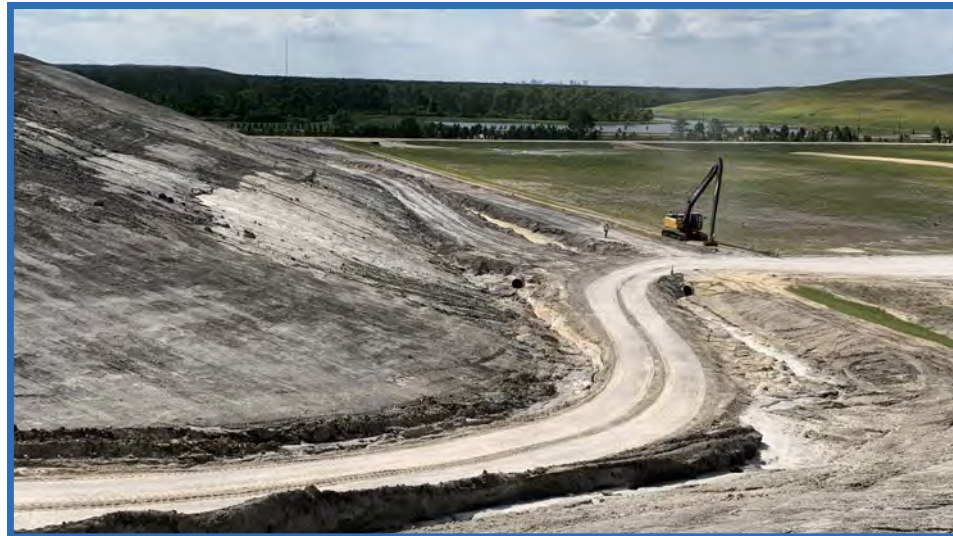
Access Ramp from West Haul Road to Western Slope of Closed Original CWSA, Looking Northwest Toward Cell 2
