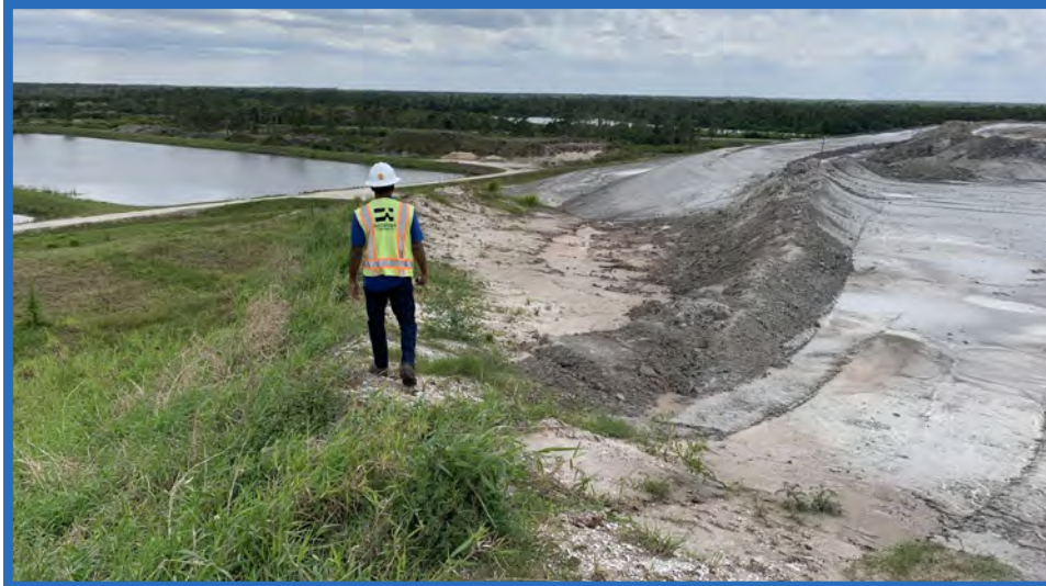
Access Ramp to Closed Vertical Expansion of CWSA and Southeastern Corner of Cell 1, Looking Southwest
