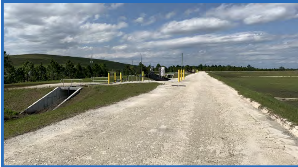
Perimeter Dike/Road West of Cell 2, Looking North
