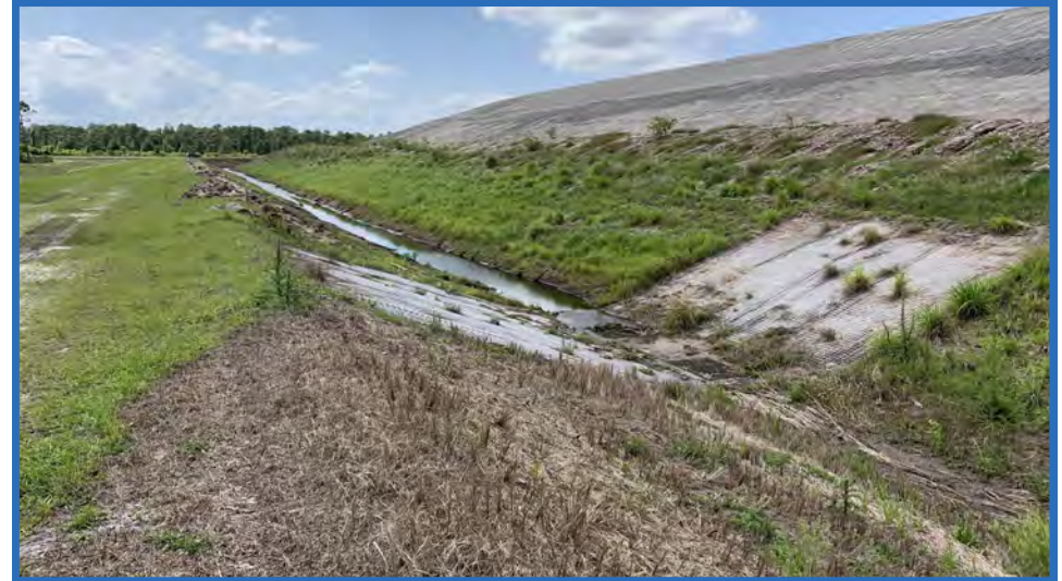
Fabriform with Inlets to Wet Detention Pond in Perimeter Ditch Around Southwestern Part of Cell 1, Looking Northwest
