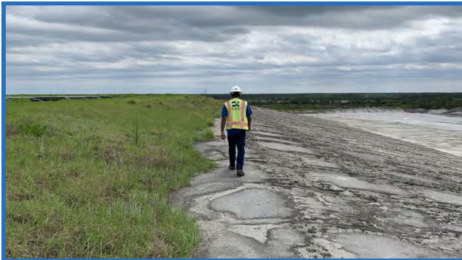
Waste Piggybacking on Western Slope of Closed Original CWSA, Looking South
