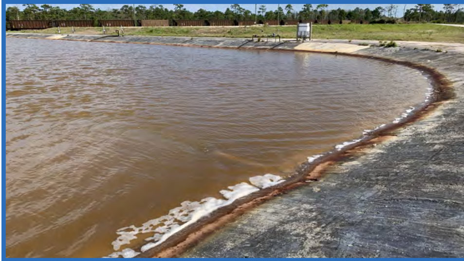
CWSA Runoff Pond South Compartment, Looking Southeast
