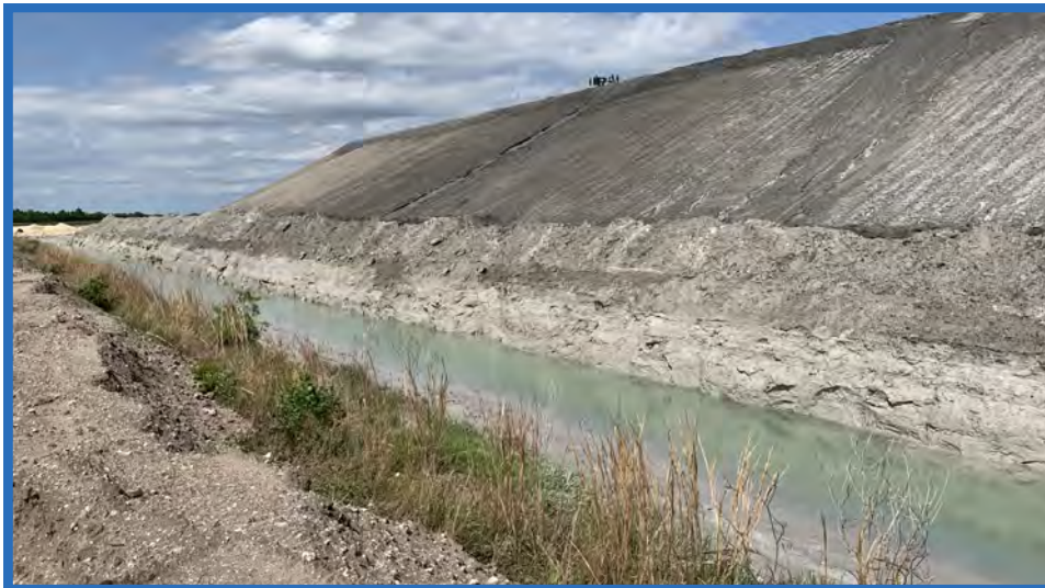
Western Slope of Waste Mound in Cell 1, Looking Northeast
