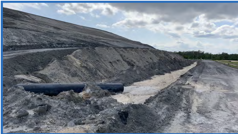
Northeastern Slope of Waste Mound in Cell 1 and Dike Between Cell 1 and Cell 2 with Temporary Culvert Under Access Ramp, Looking West
