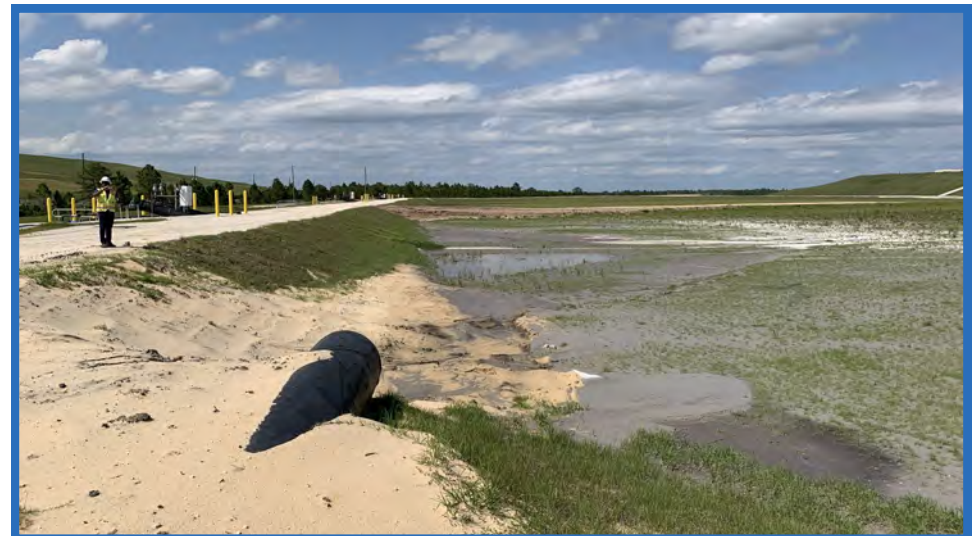
Cell 2, Looking North
