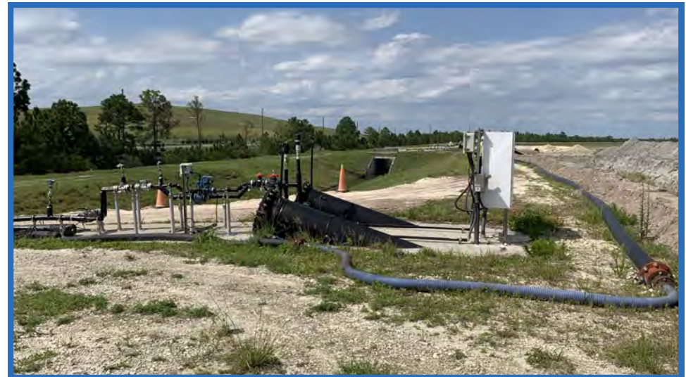
Connection of Discharge Pipeline from Auxiliary Pumps to Leachate Force Main via Pump Station
