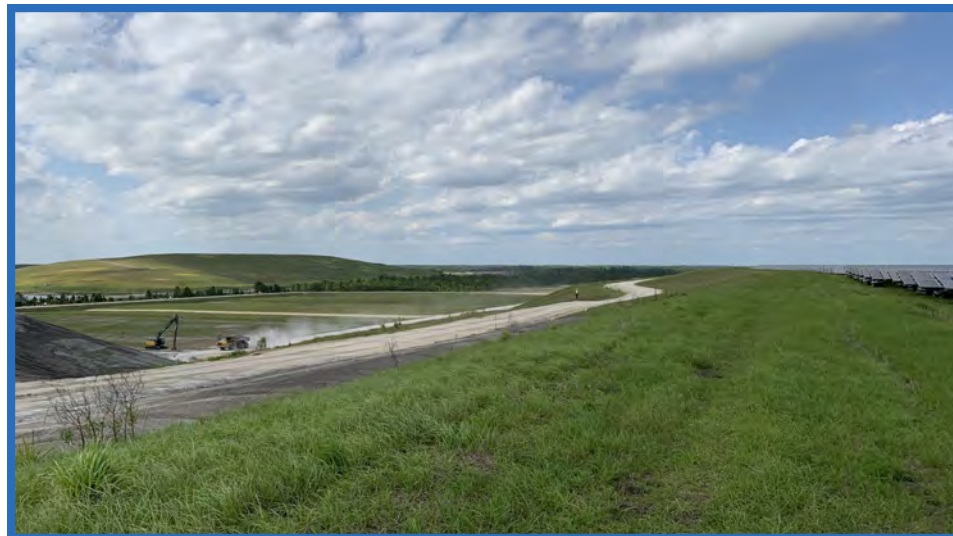
Closed Vertical Expansion of Original CWSA, Looking Northwest
