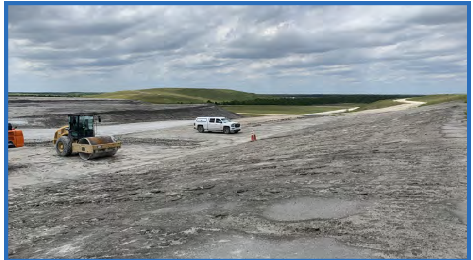
Waste on Western Slope of Closed Original CWSA, Looking Northwest Toward Cell 2
