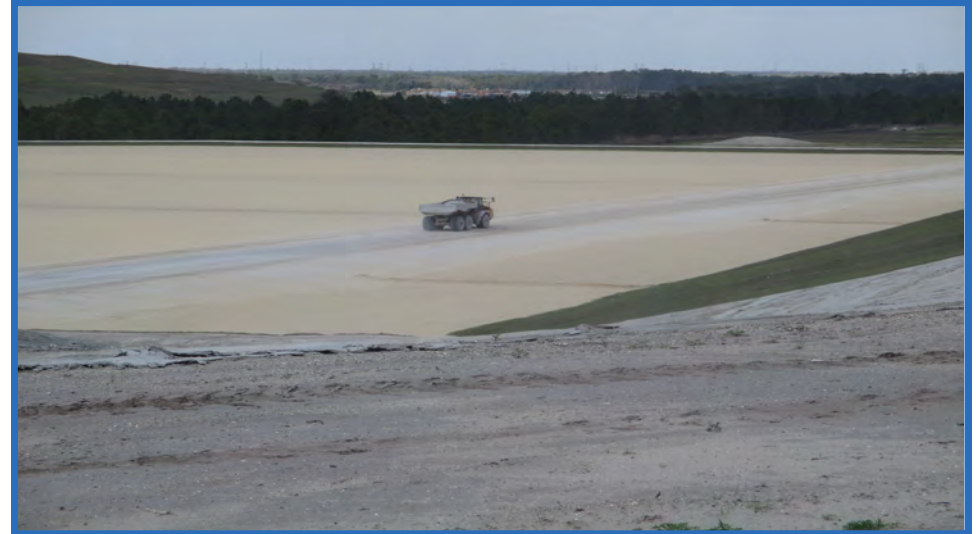
West Haul Road through Cell 2 Looking Northwest
