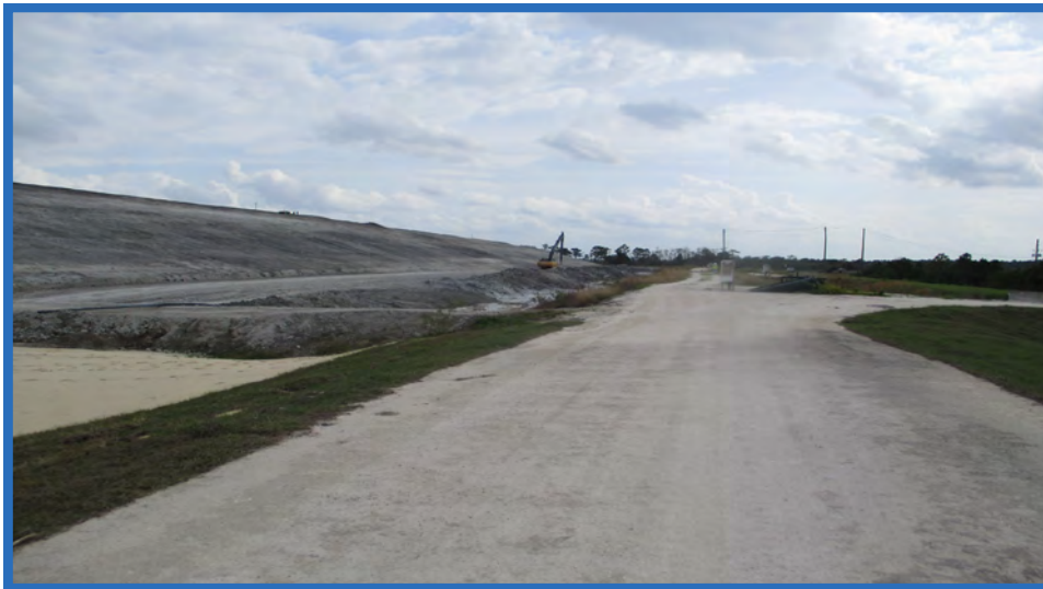
Waste Mound and Containment Dike Looking South
