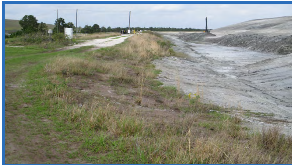
Western Side of Cell 1 Looking North from South of Sump 1
