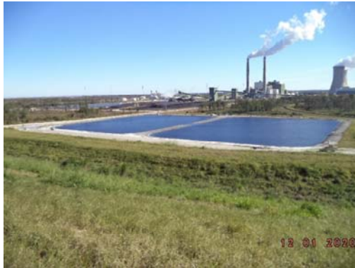
CWSA Runoff Pond
