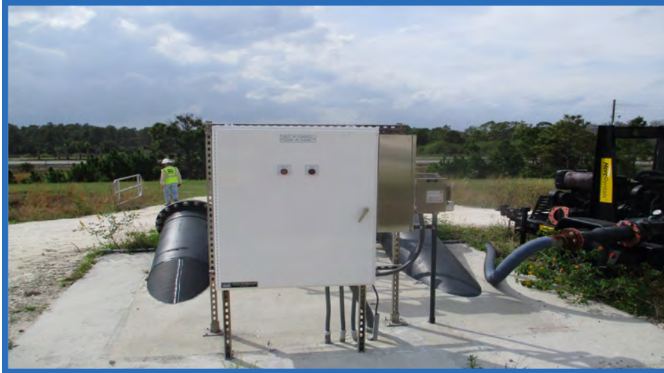
Replaced Control Panel and Pump Station for Sump 2
