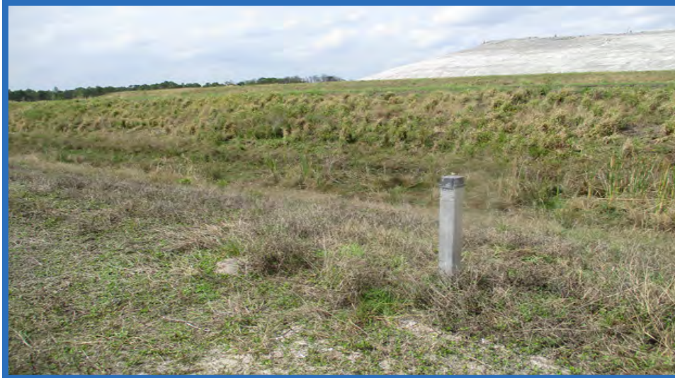
Monitoring Well MW-10
