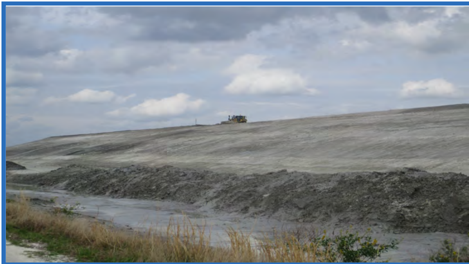
D6N Dozer Grading Waste in Southeastern Part of Cell 1 Looking Northeast
