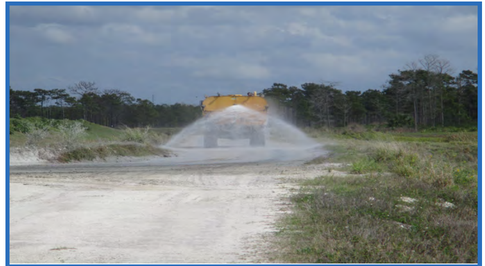
Dust Control Measure along East Haul Road Looking East
