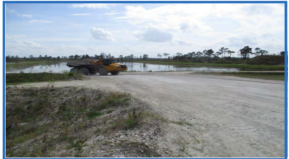
Articulated Dump Truck Hauling Waste through East Haul Road for Placement in Cell 1
