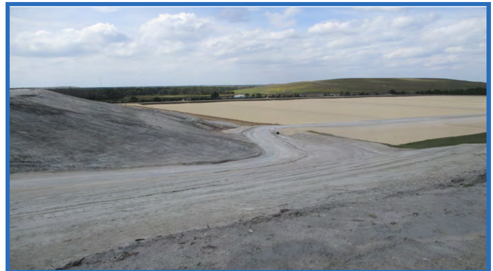
North Cell 1 Access Ramp through Cell 2 Looking Northwest
