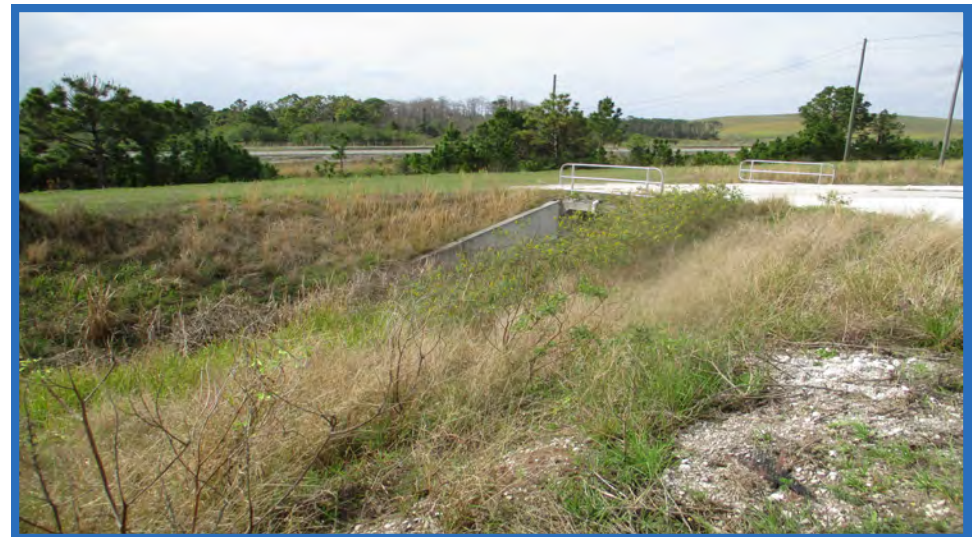
Stormwater Ditch with Box Culvert and Access Road on the Western Side of Cell 1, Looking Northwest
