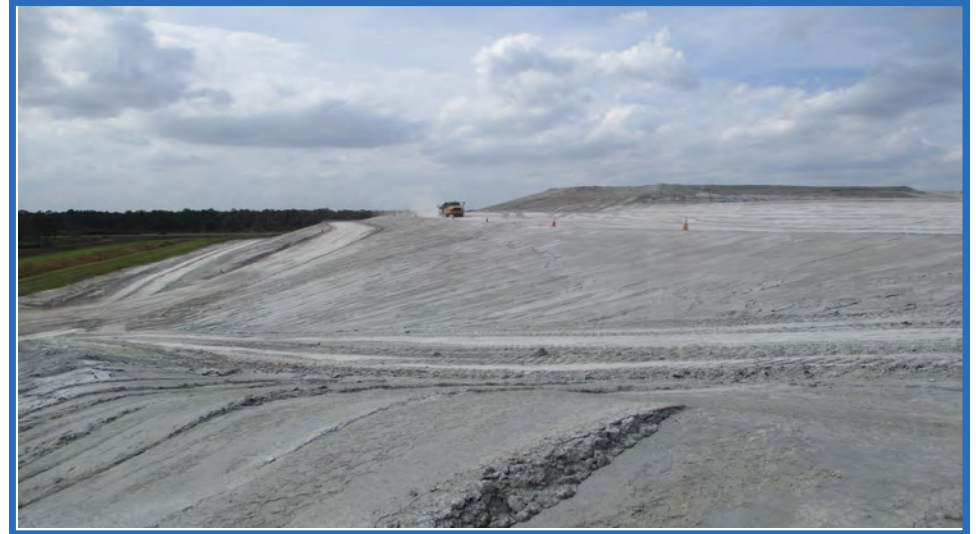
Waste in Southern Side of Cell 1 with Access Road Looking West
