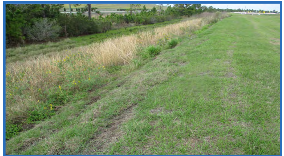
Cell 1 Perimeter Dike Looking North
