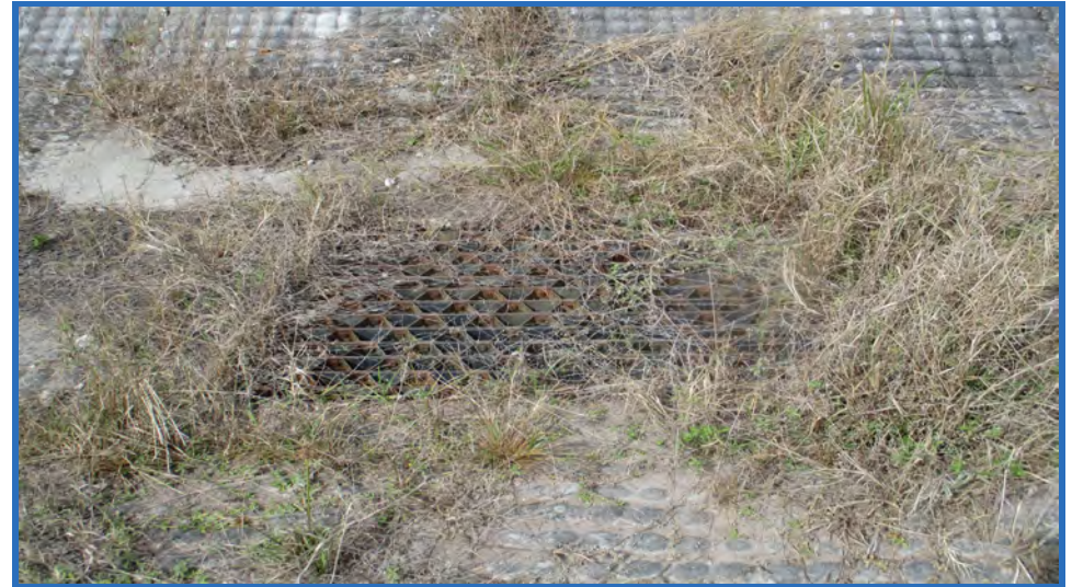
Inlet Box Connected to Pipes Discharging to Wet Detention Pond
