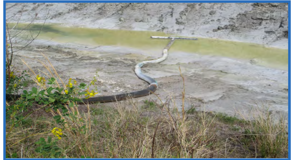
Intake Pipeline for Auxiliary Pump in Preceding Photo
