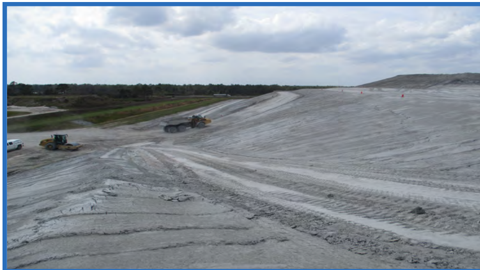
South Cell 1 Access Ramp Looking West
