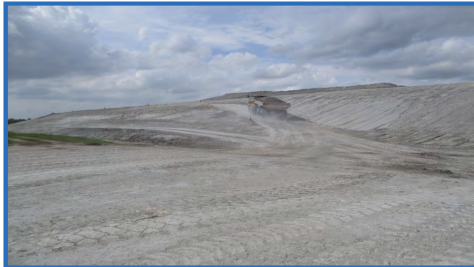
Access Ramp Through Waste Mound in Cell 1 Looking Northwest
