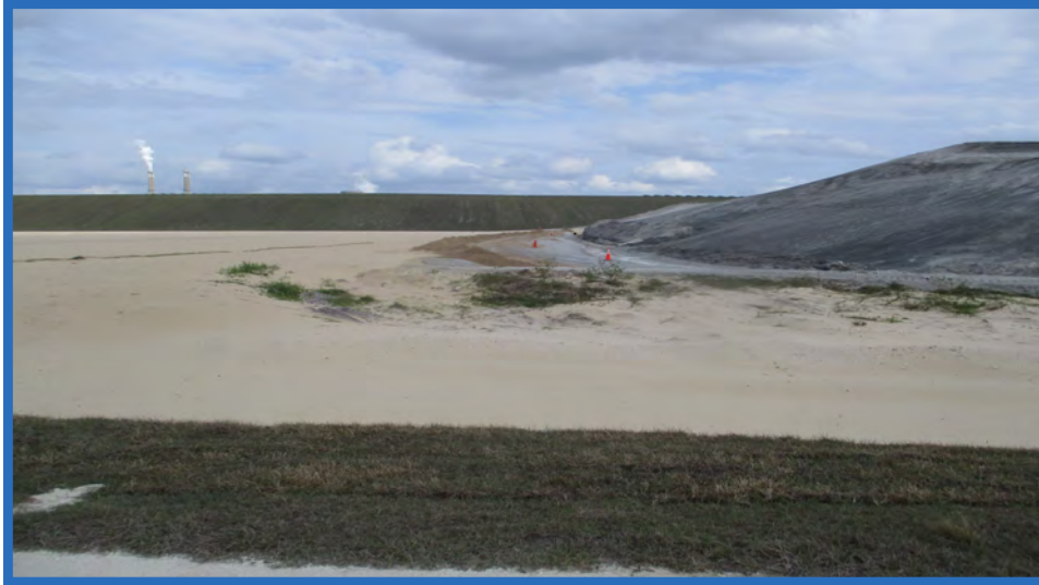
Recently Constructed Cell 2, Divider Dike, and Waste Mound in Cell 1 Looking East
