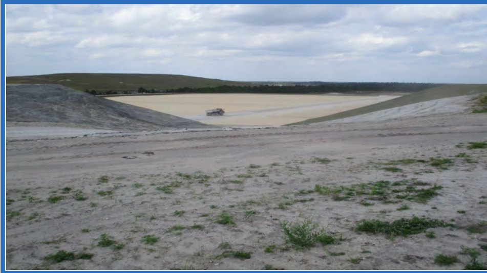
Cell 1 Waste Mound and Recently Constructed Cell 2 Looking Northwest from Reverse Bench
