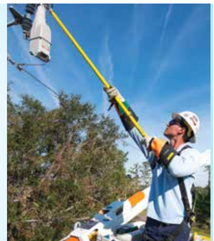
Roger McBride, Line Technician, installs a TripSaver II device on a test line at the Pershing Operations Center.
