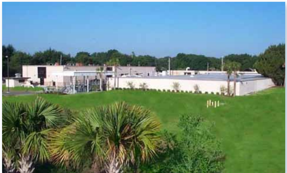
CWF Water Facility
