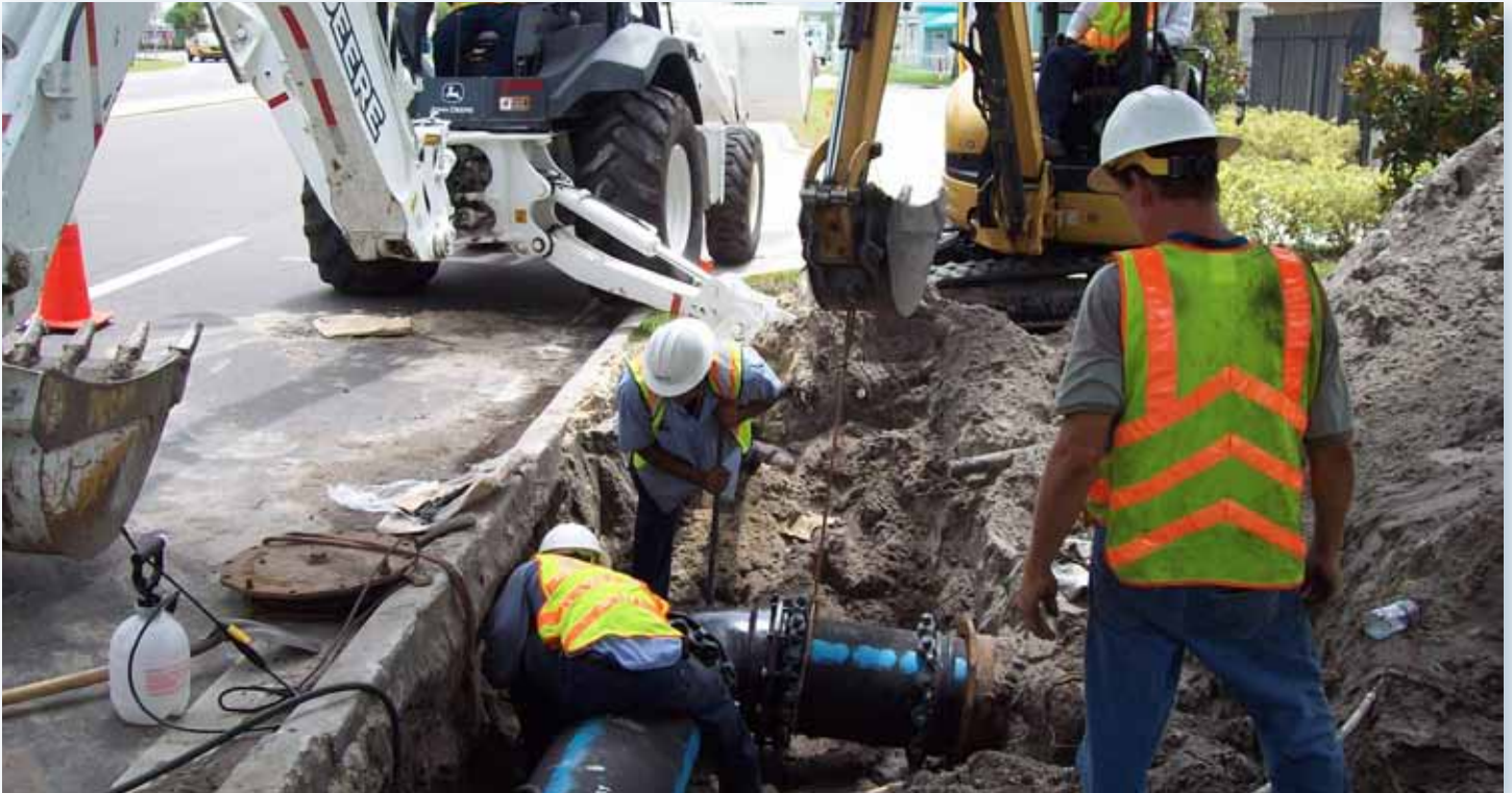
WDIS crew performed repairs on Robinson Street water distribution system
