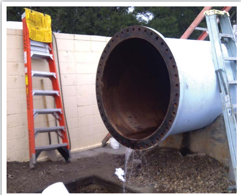
48-inch pipe repair at Sky Lake Water Treatment Plant
