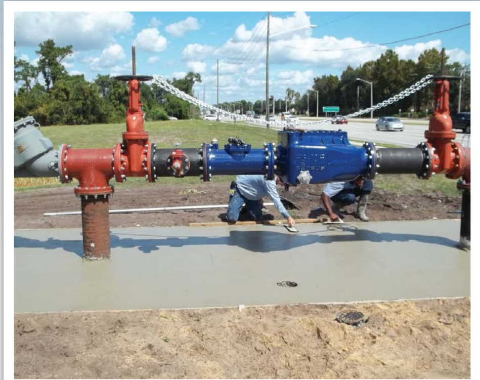
10-inch sensus Omni meter at Valencia College on Kirkman Road
