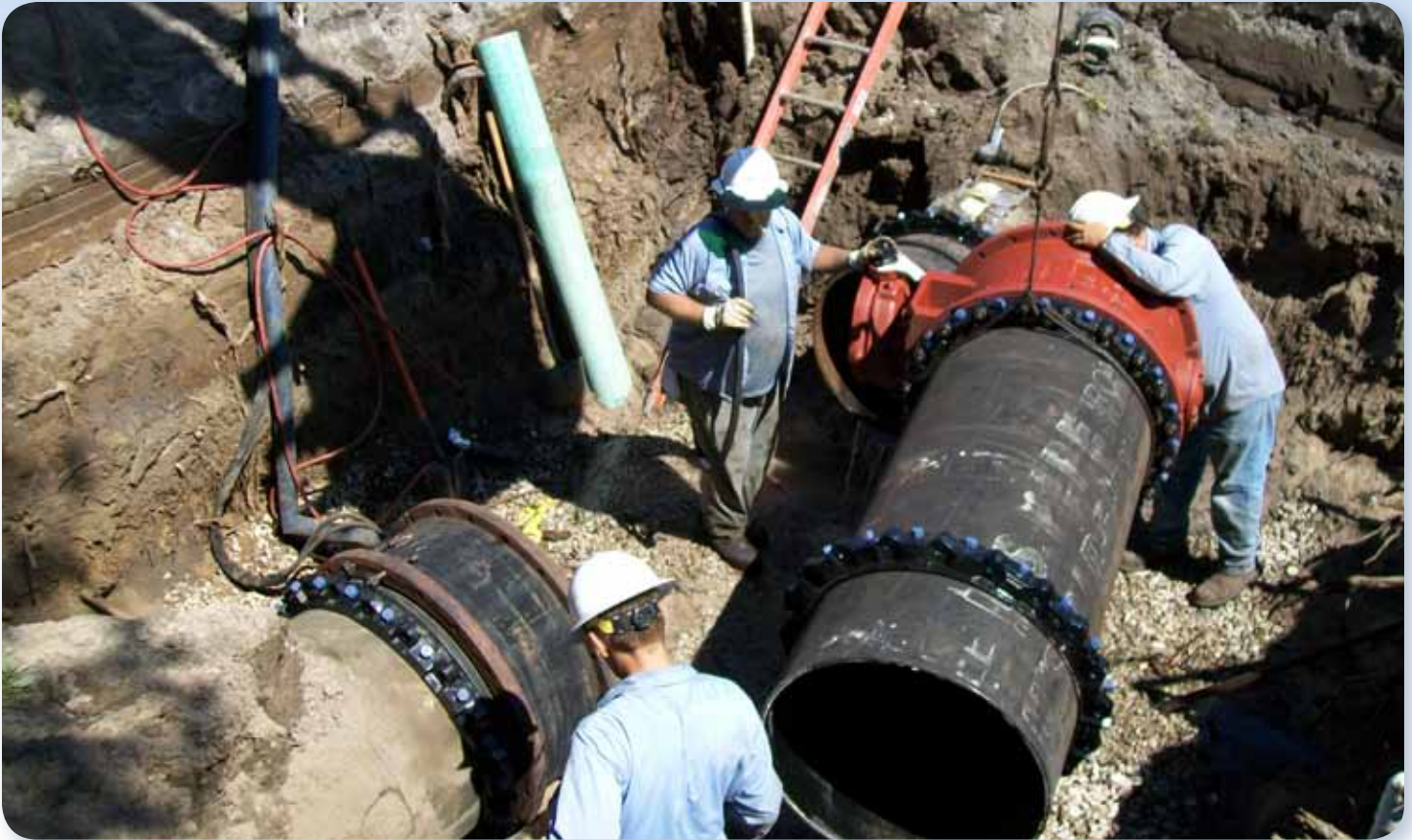
Installing 30" Valve at Kirkman Water Plant
