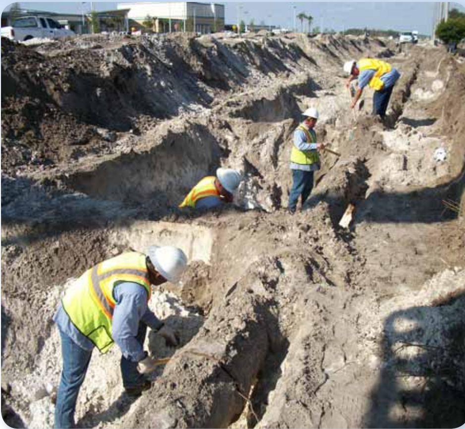
Narcoossee pipe lowering
